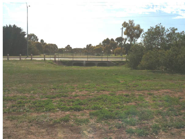
Figure 5.4: Culverts under Derrimut Road allowing high flow outlet from the D1 Drain Reserve
