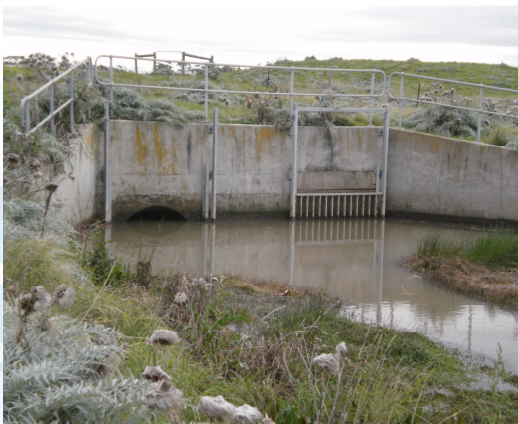
Figure 5.11: The siphon allowing the D1 Drain to flow under the Western Trunk Sewer
