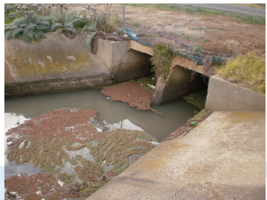
Figure 5.12: The siphon allowing the D1 Drain to flow under the Historical Western Outfall Sewer
