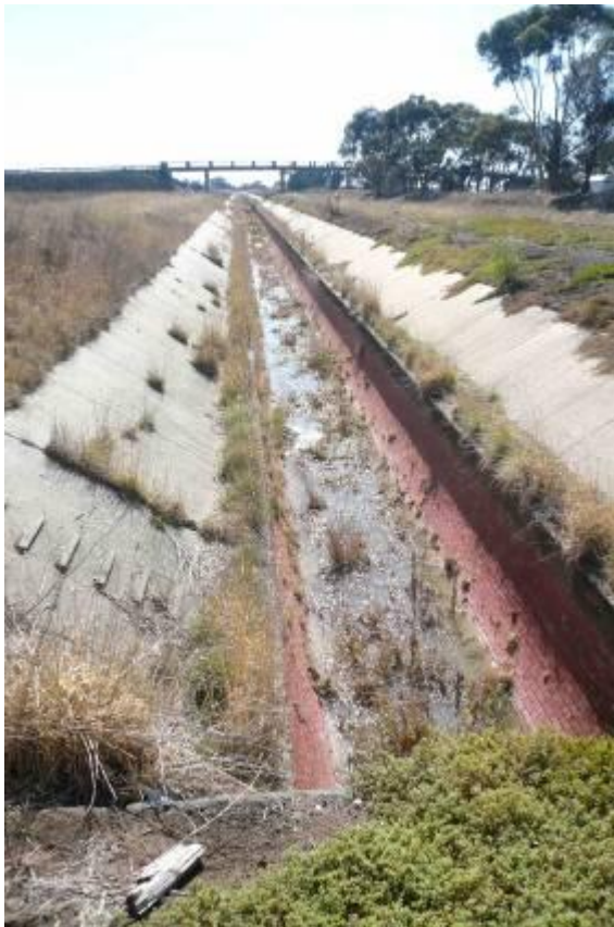
Figure 19 Section of the Main Outfall Sewer running through the subject site as an open brick-lined channel.
