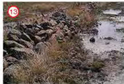
Existing dry stone wall (substantial) - to be retained
