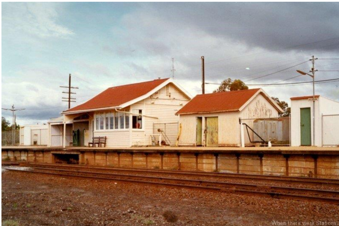
Figure 15: Former Rockbank Station and signal box buildings, 89
