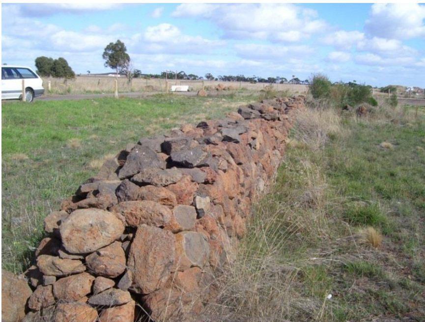
Figure 46: Conserved dry stone wall near Hopkins Road (east of study area)
