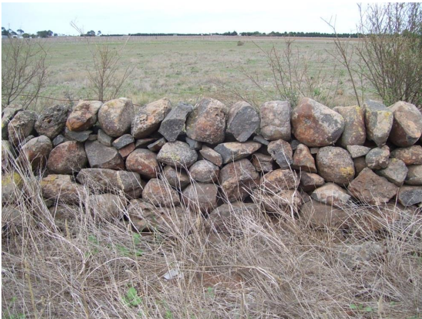
Figure 44: Detail of dry stone wall on east side of Leakes Road
