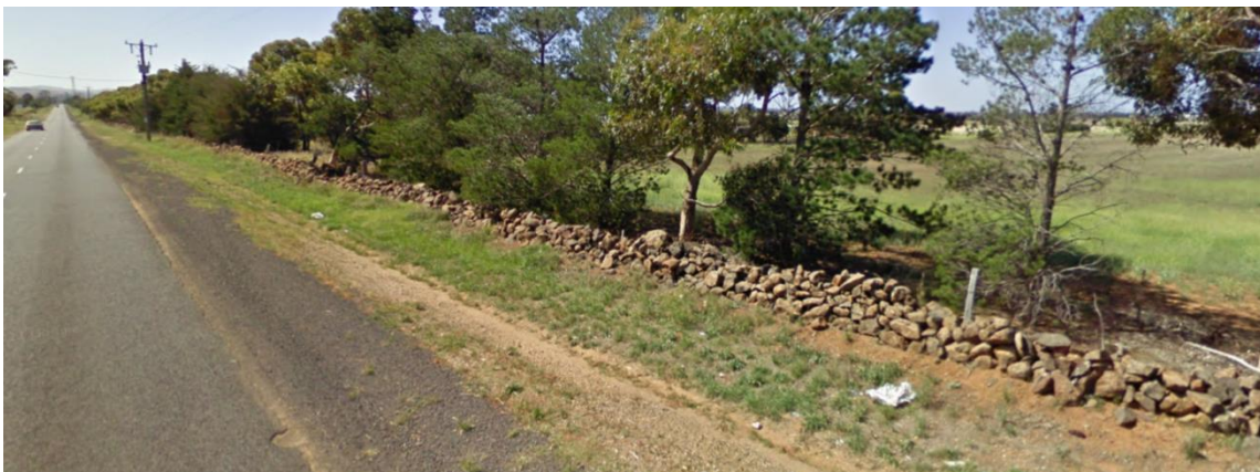
Figure 43: Dry stone wall at moderately intact wall on east side Leakes Road
