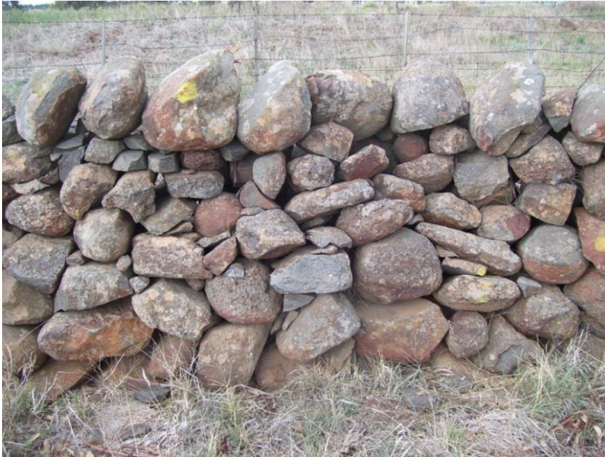
Figure 45: Detail of dry stone wall south side Greigs Road
