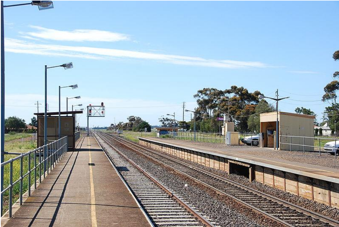
Figure 32: Rockbank Railway Station
