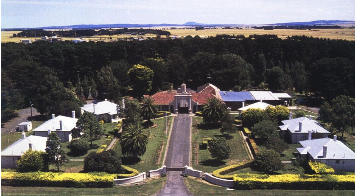
Figure 22: Australian Wireless Beam Station. 108
