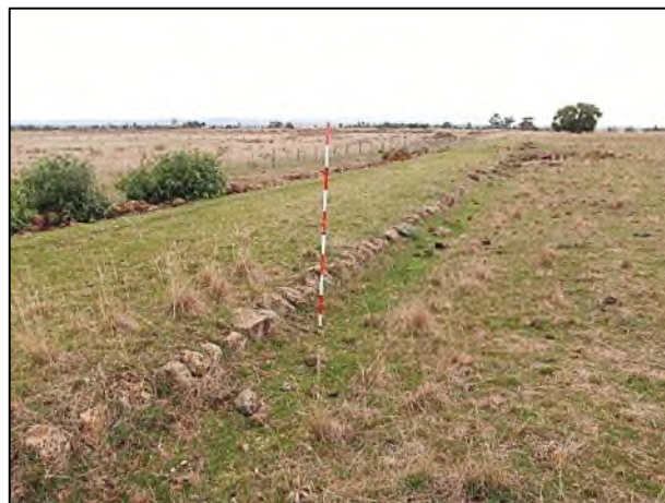
Plate 34: The stone embankment lining and spoon drain on the eastern side near the southern end (Prop Ref #41)
