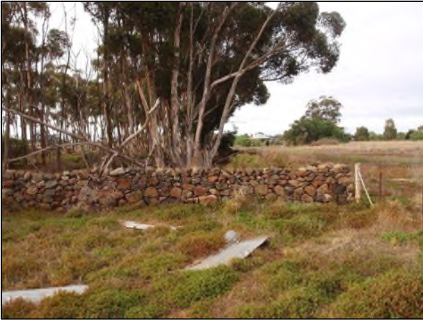
Plate 10: Single or double dry stone wall on Deanside (Property Ref #14).
