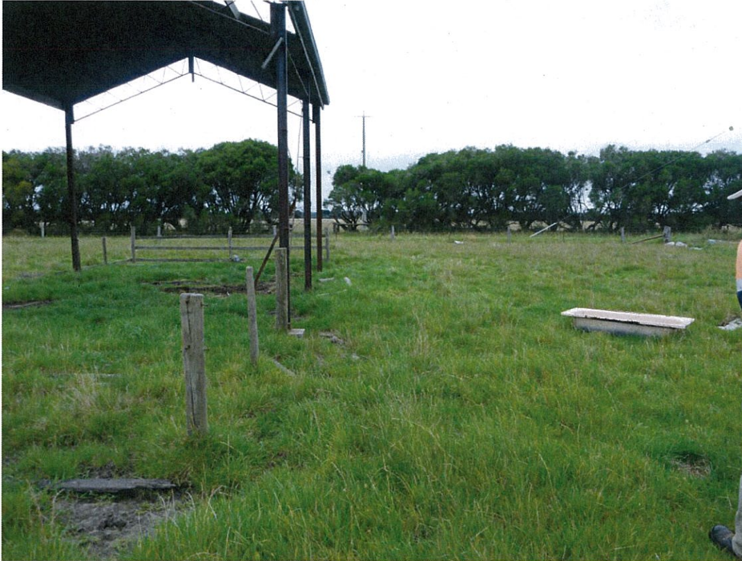
Photograph 19: View of debris surrounding shelter located south east corner of site. Debris included bath tub, galvanized iron, timber, brick, concrete, tyres and asphalt.
