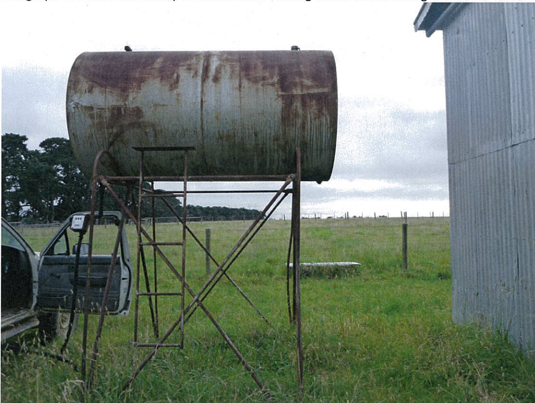
Photograph 16: Above ground storage tank (AST) containing diesel. This AST was still in use.
