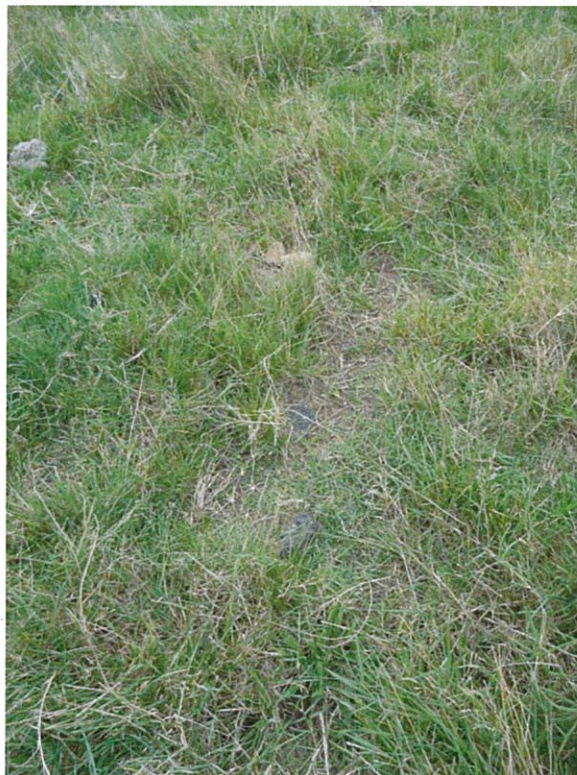
Photograph 18: View of pieces of concrete, brick and asphalt along the south boundary in between the dammed water course and Smiths Lane.
