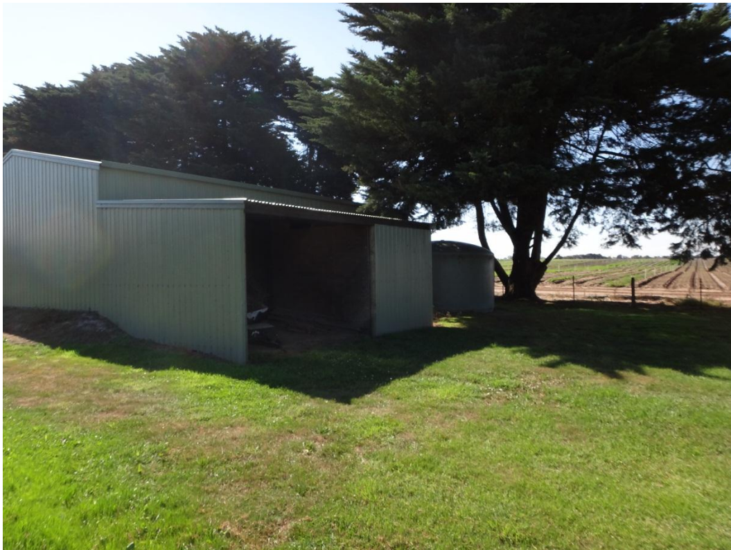
Photograph 102: Wood and vehicle storage shed to the north east of the residence.
