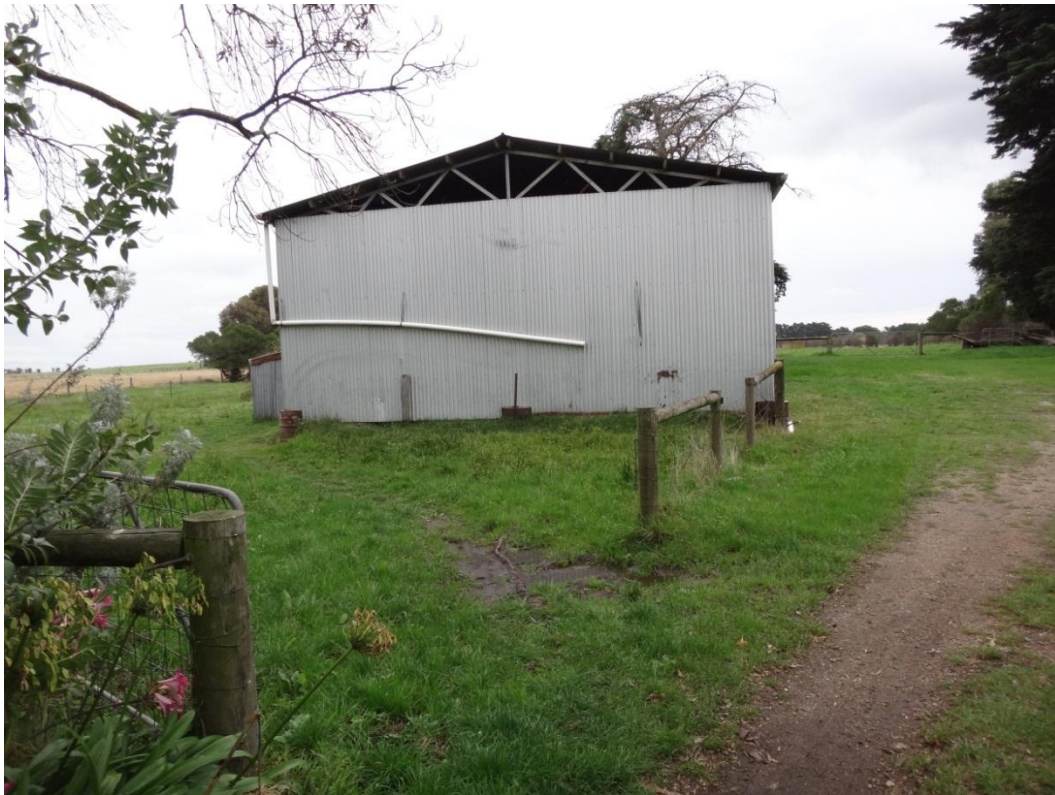
Photograph 11: View south of hay shed.
