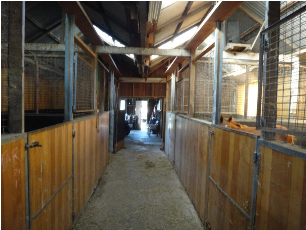
Photograph 41: Horse stables in north east portion of the property.
