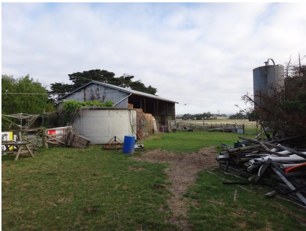
Photograph 39: Storage area to the east of the former milking shed and residence.
