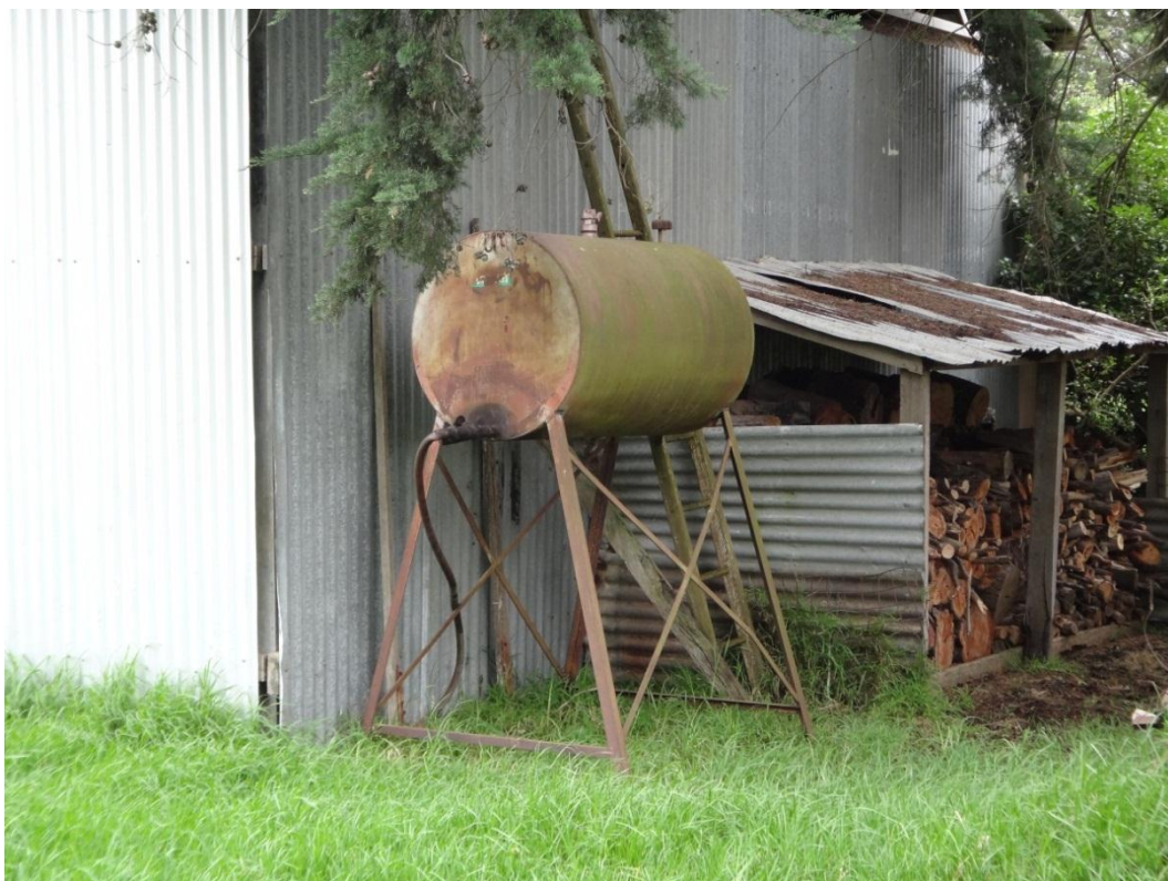
Photograph 13: Diesel AST located along the south wall of the hay shed.
