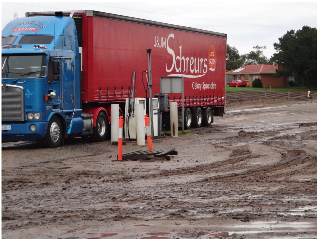
Photograph 134: Refuelling bowsers linked to diesel USTs.
