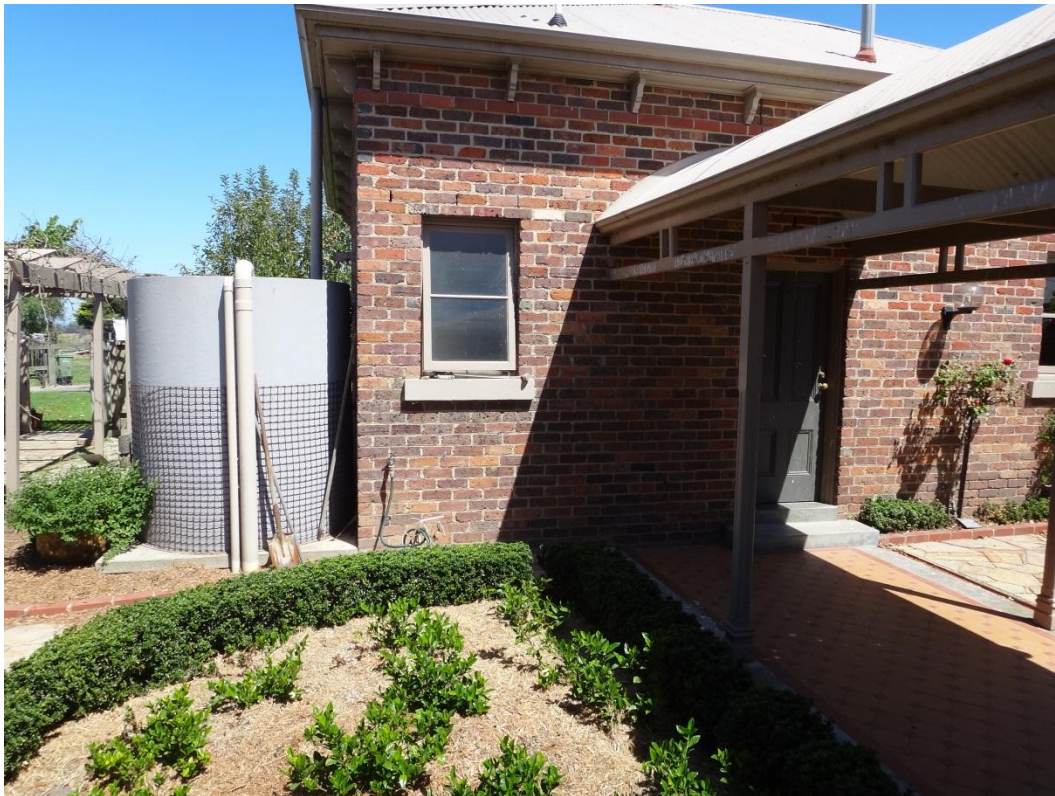
Photograph 105: Brick residence and garage in the west portion of the property.
