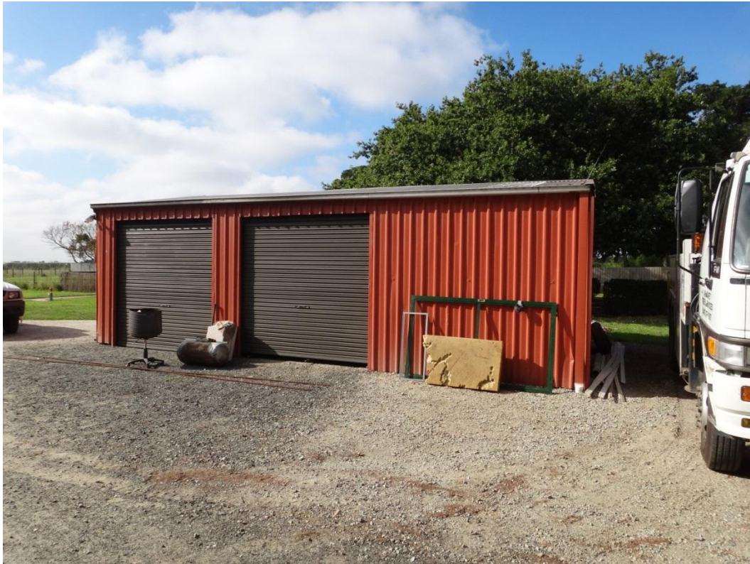
Photograph 46: Storage shed/entertainment room north of residence.
