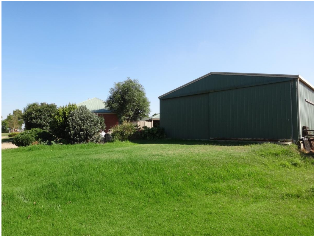
Photograph 94: Storage shed along east property boundary.
