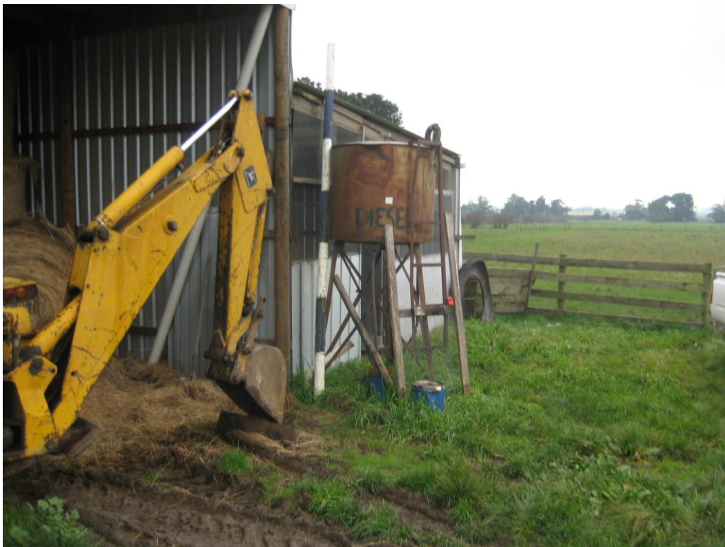
Photograph 148: Diesel AST located adjacent to a hay shed in the west portion of the property.
