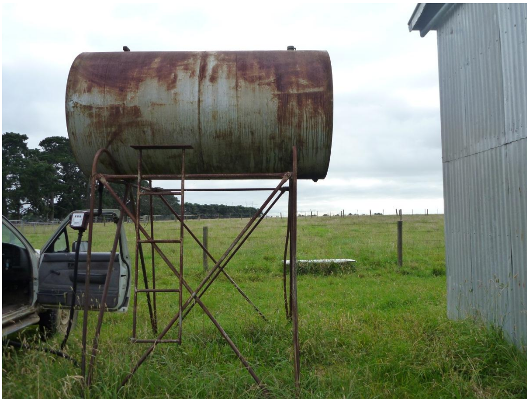
Photograph 25: AST located north of former milking shed.
