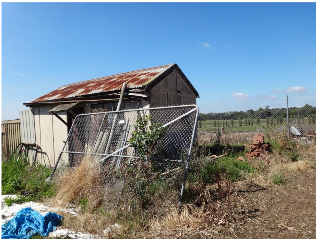
Photograph 60: small storage shed located in the south portion of the site.
