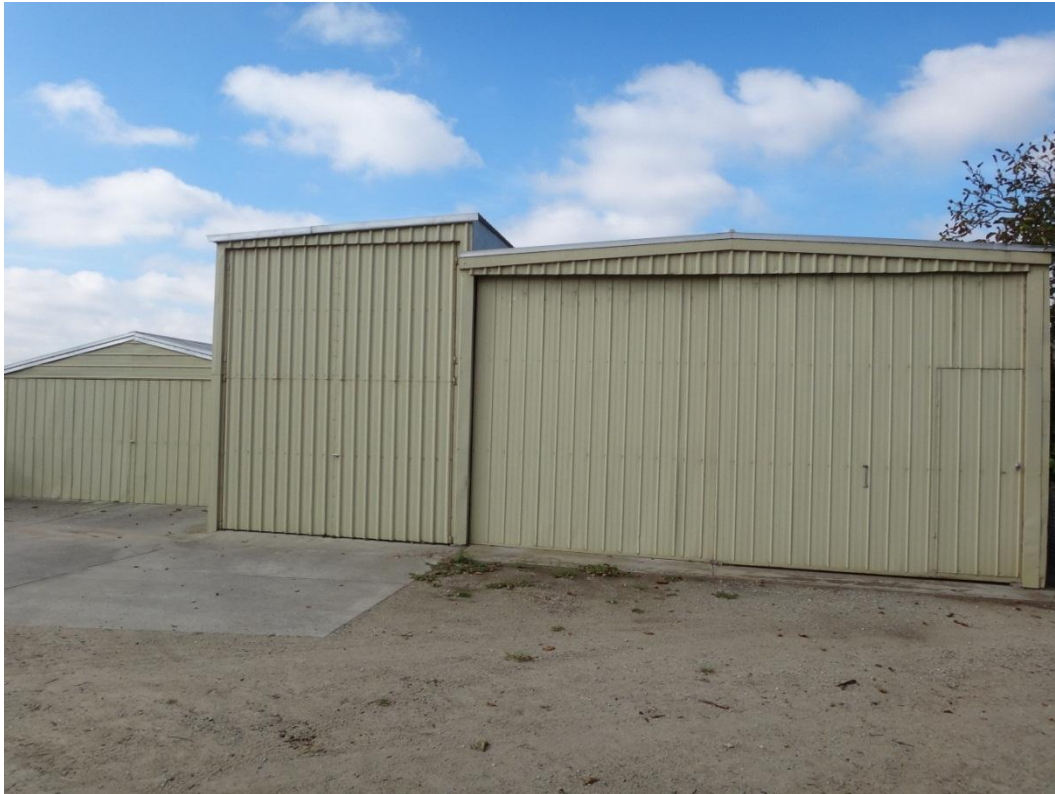
Photograph 68: Farm machine storage.
