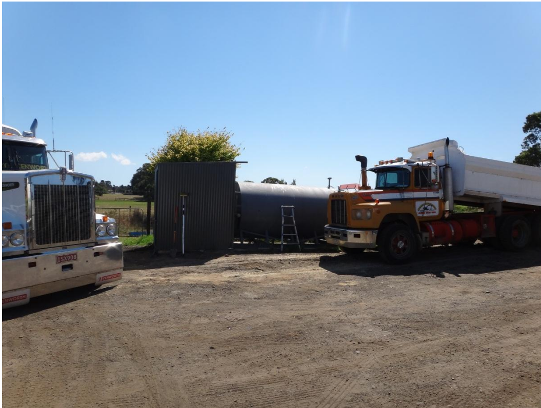
Photograph 123: Truck parking and refuelling in the west portion of the property.
