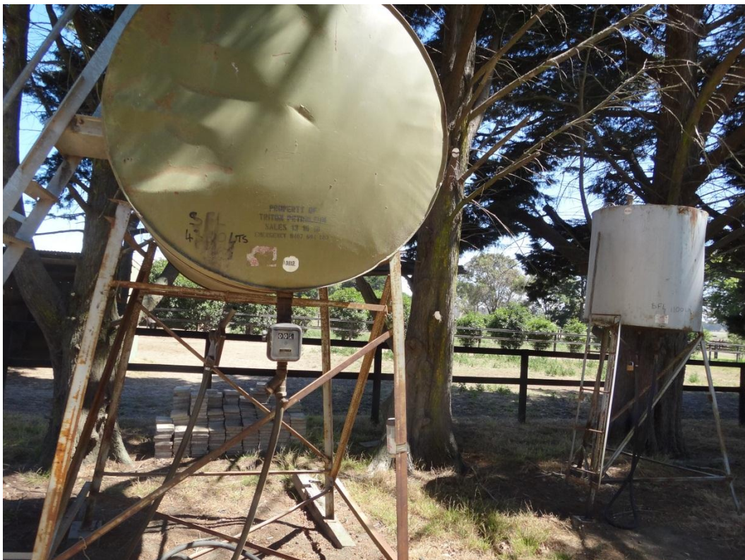
Photograph 87: Two diesel ASTs located to the north of the stables.
