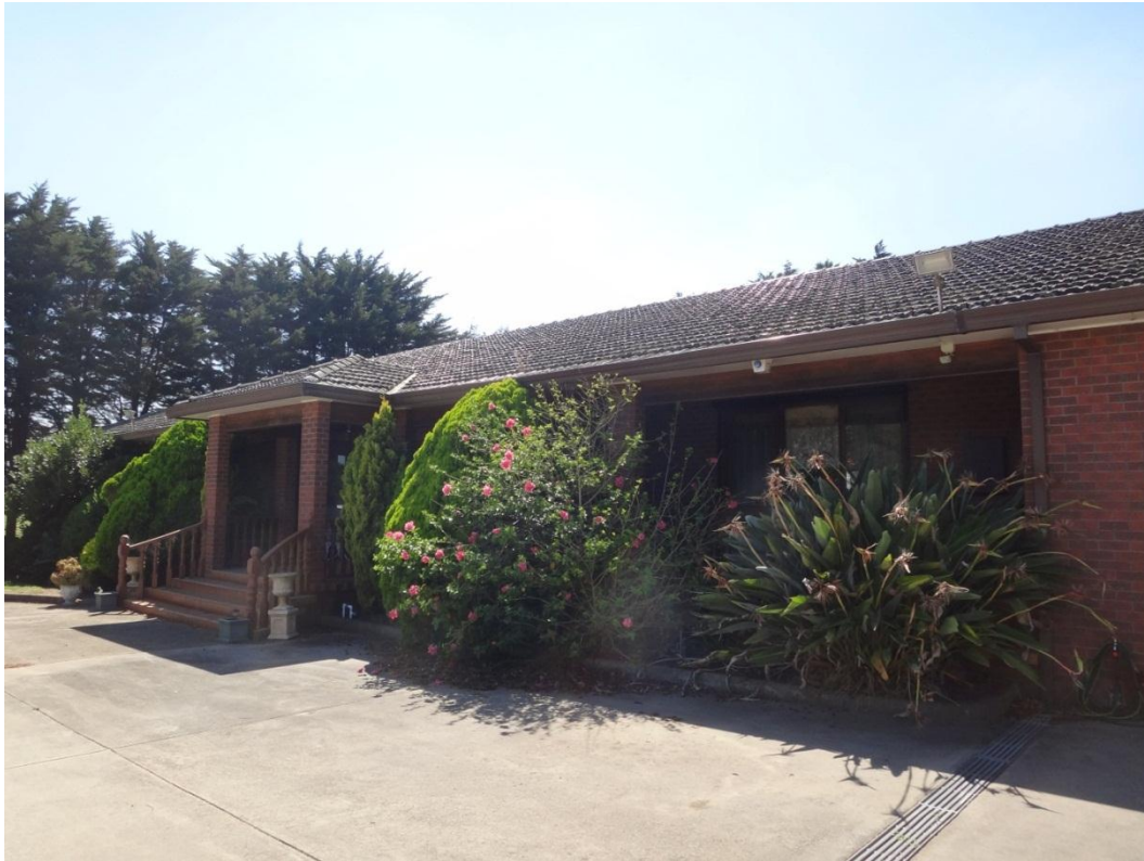
Photograph 55: Concrete driveway and brick residence.
