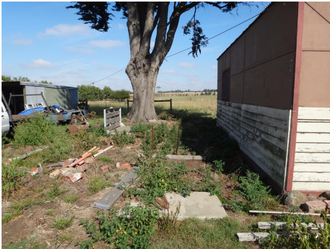
Photograph 54: Area of disturbance/demolished building west of residence.
