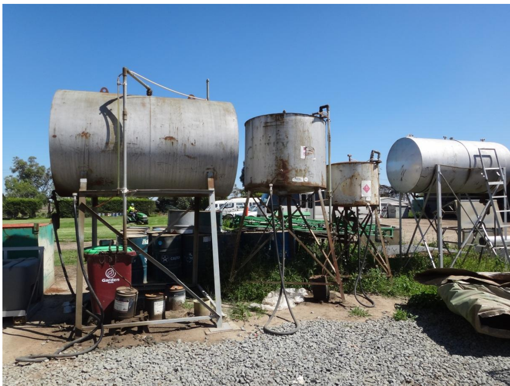
Photograph 128: ASTs located to the north of the vehicle maintenance shed.
