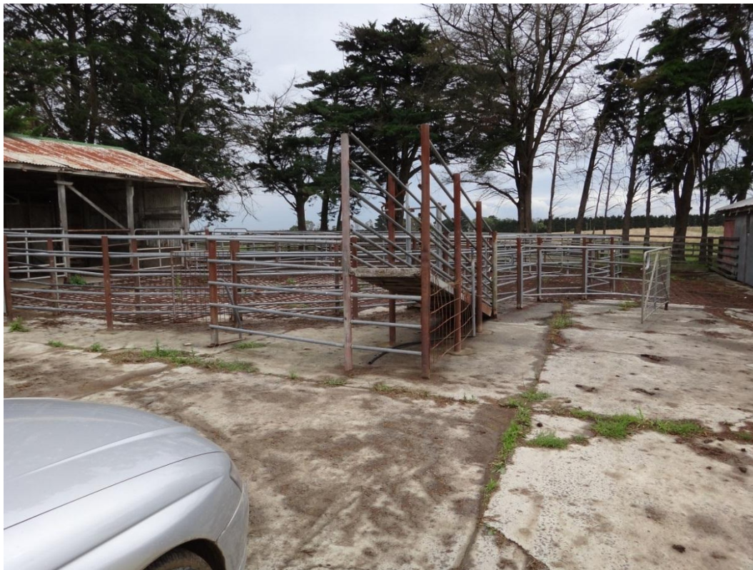
Photograph 22: Milk shed stock pens and loading ramp.
