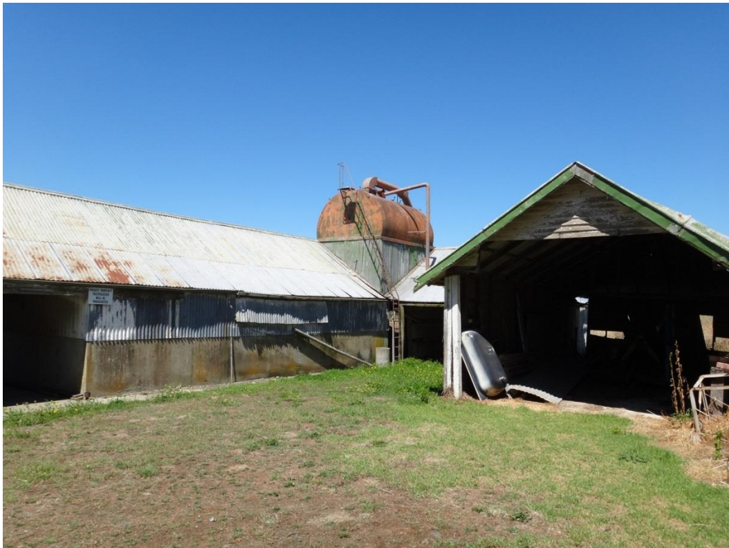
Photograph 76: Former milking shed with water storage tank on the roof located to the south of the residences.
