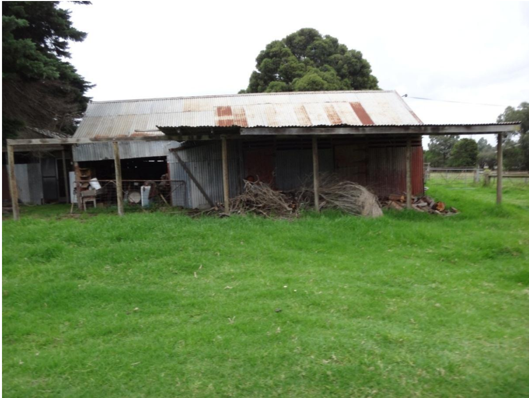
Photograph 10: View west of old farm/storage shed.
