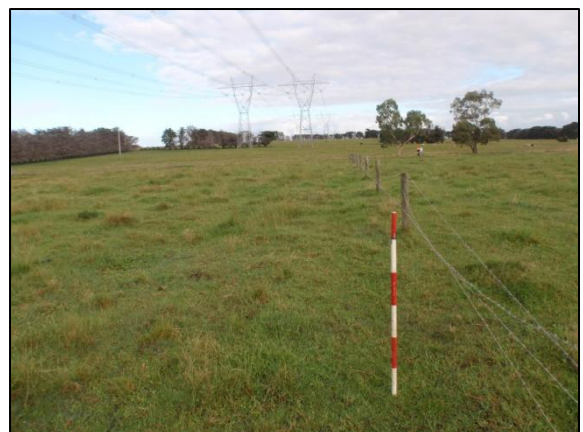
Plate 10: Power transmission easement, facing west
