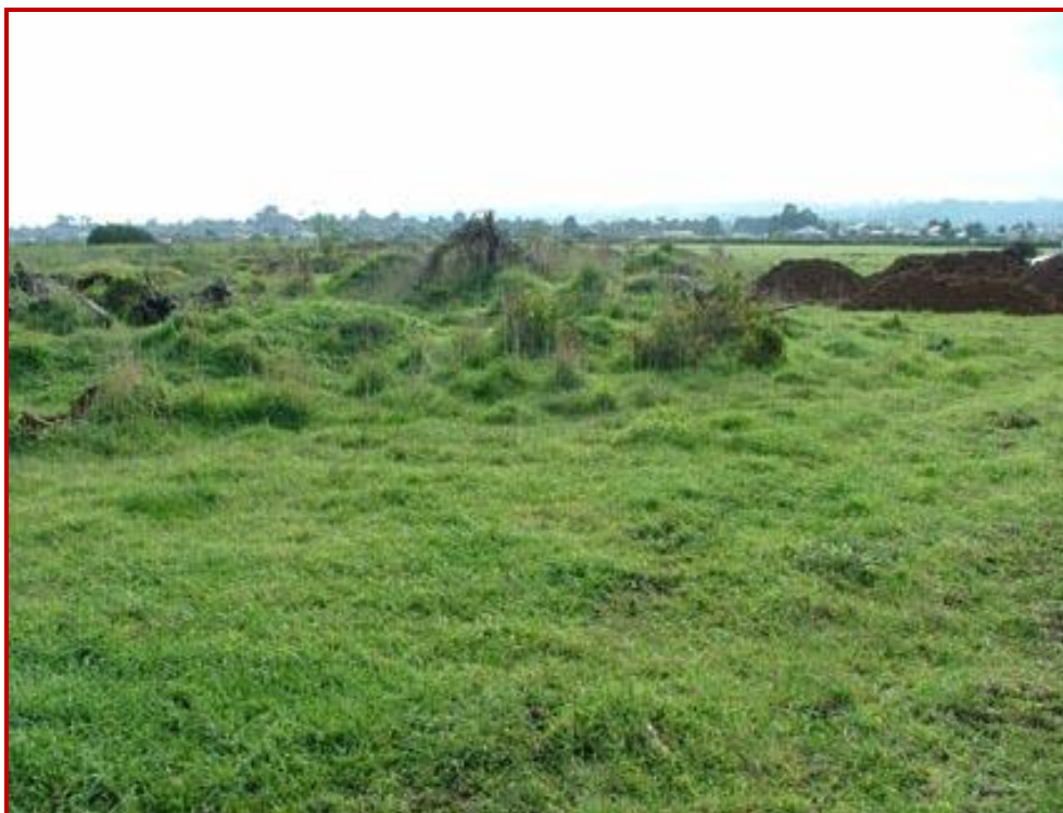
Figure 21 – Fill platform and recently deposited spoil.
