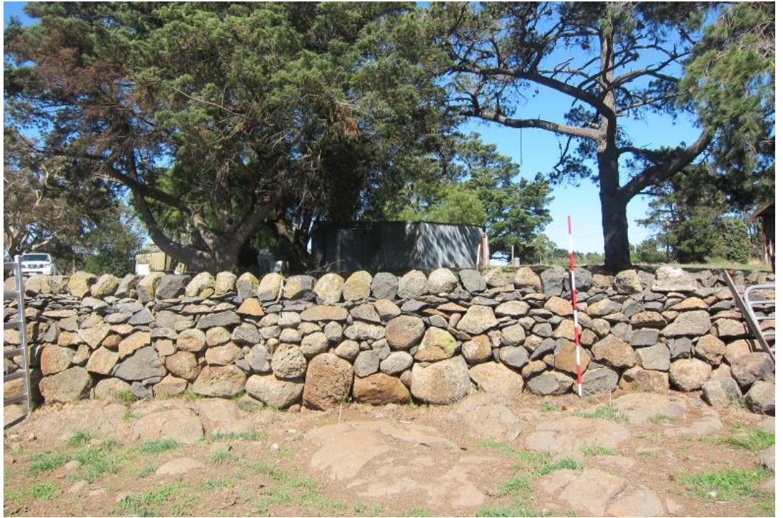
Figure 5 - Technically refined dry stone wall to the north of the house, looking south.
