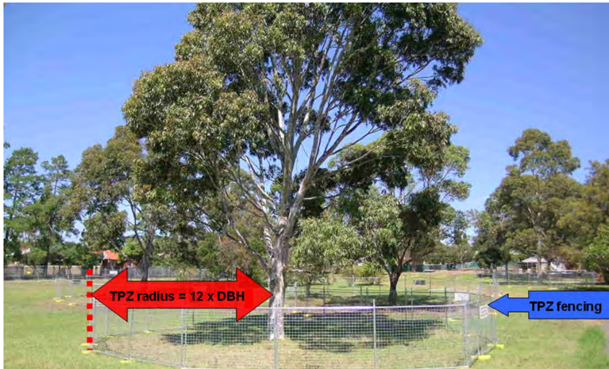
Figure 16: TPZ fencing is erected around retained trees prior to site works.
