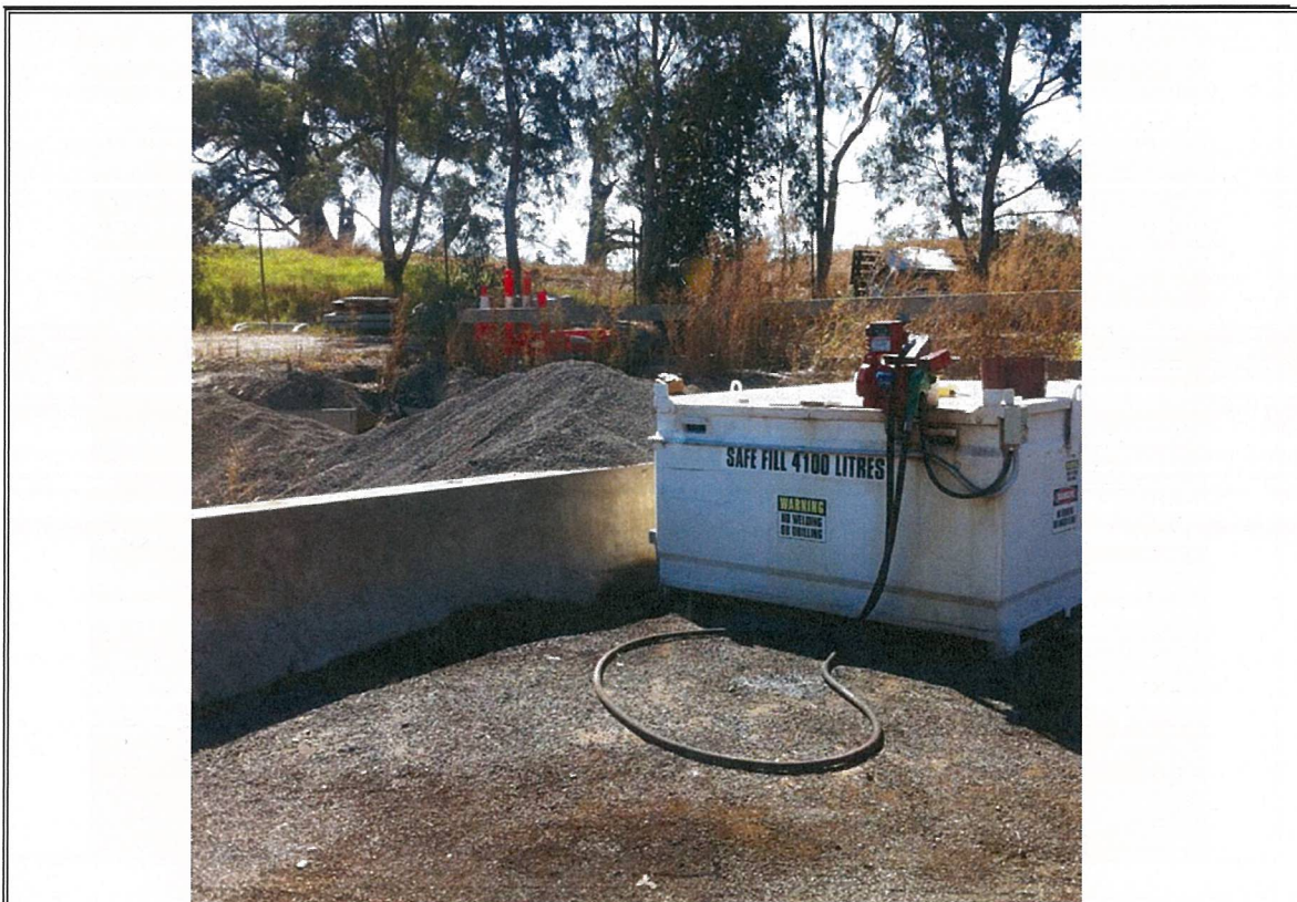
Photograph 5. Evidence of staining next to the diesel AST (785 Cranbourne-Frankston Rd)
