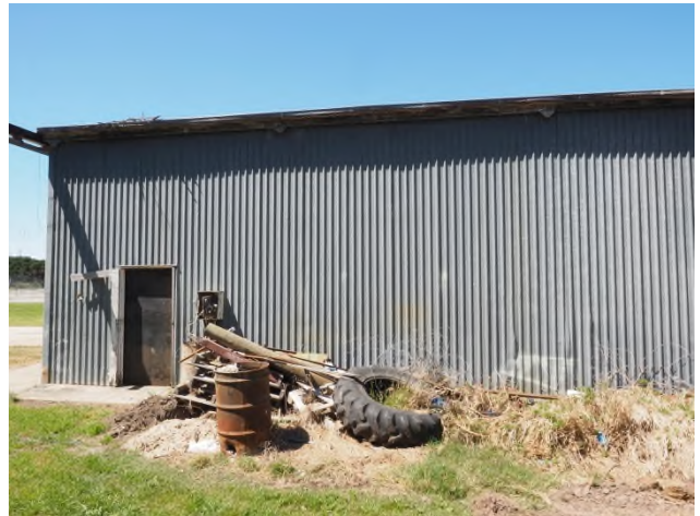
Plate 4: Galvanised steel IBR sheeting on the northern side of Building 1, facing south
