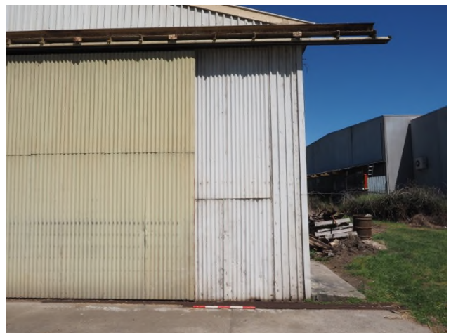
Plate 6: Detail of the door leaves and slide-rails in Building 1
