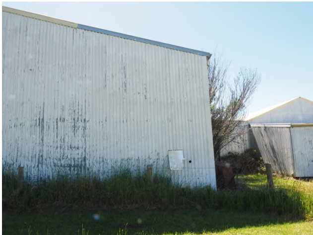
Plate 3: Corrugated steel cladding on the rear elevation of the building, facing east. Note the small fan-outlet off the 'quarantine room'
