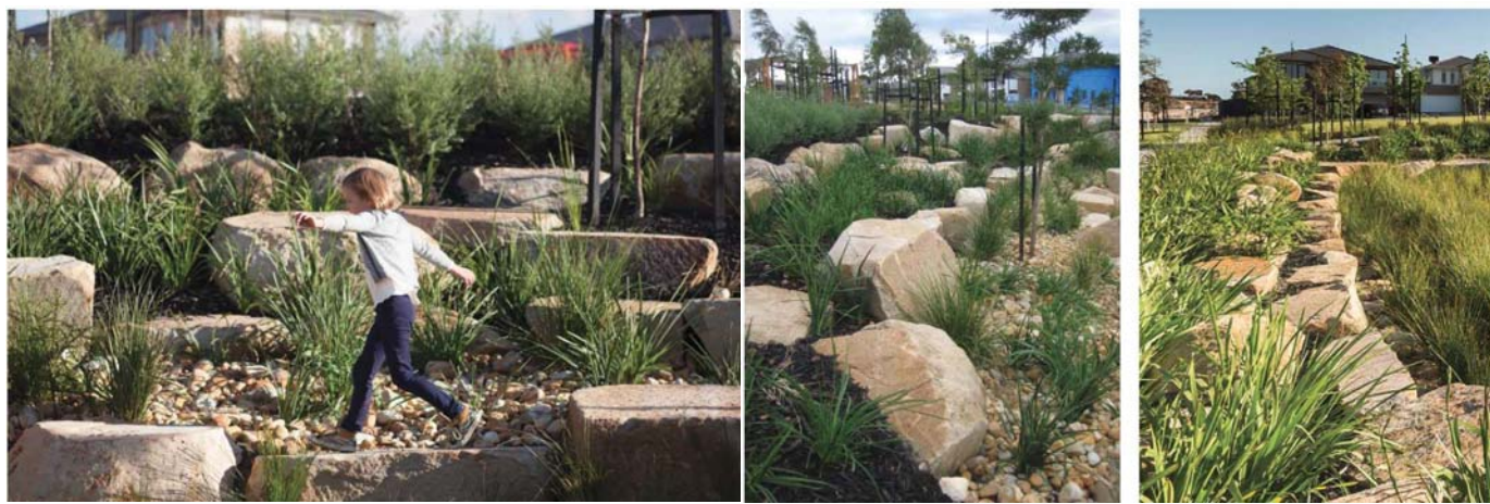
Figure 3.21 – Planted rock stabilized batters offer flexibility with slopes and a more diverse landscape.
