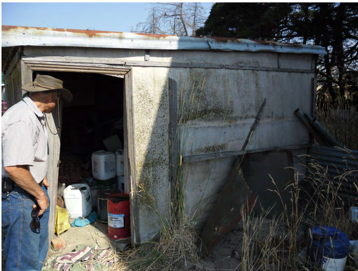
Photograph 21 – Chemical storage shed with asbestos cement sheet walls, 2040 Mickleham Rd (facing north)
