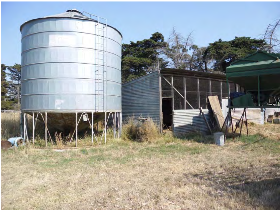
Photograph 02 - Poultry shed and feed silo at 2040 Mickleham Rd (facing NW)
