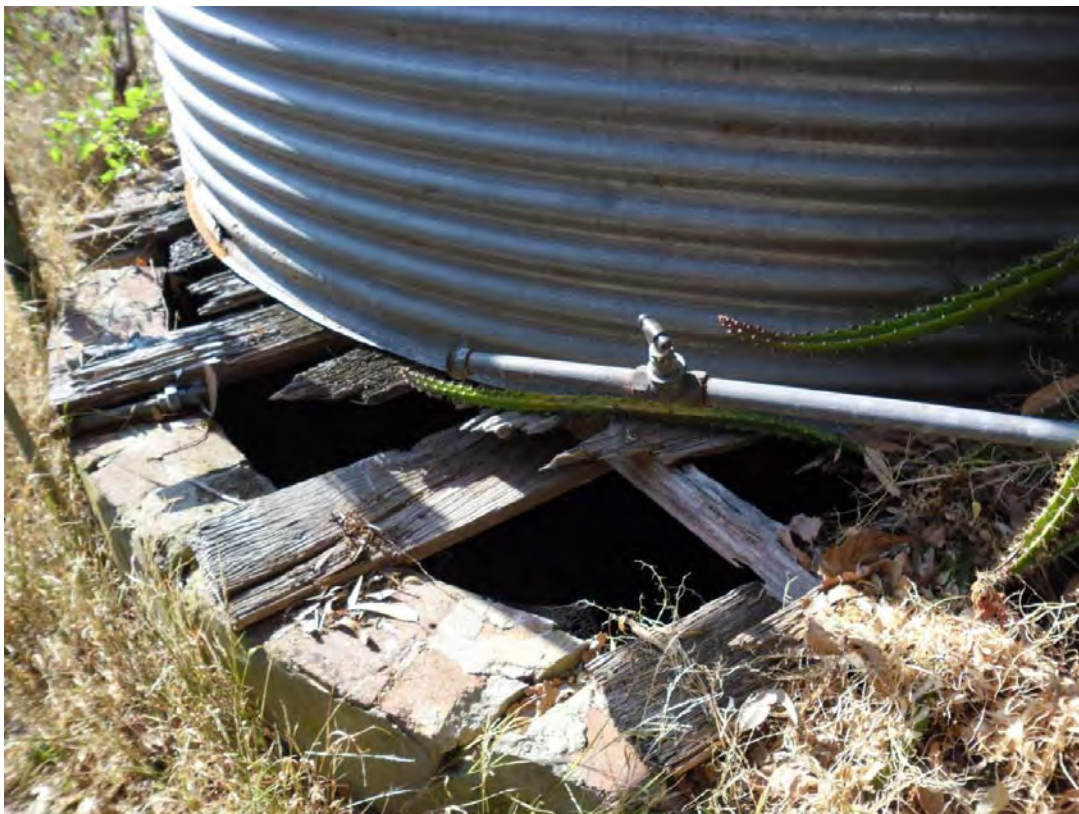
Photograph 08 - Open well adjacent to septic tank, 2040 Mickleham Rd (facing east)
