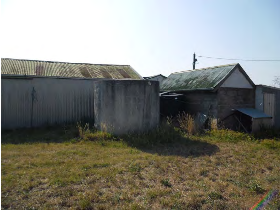
Photograph 03 - Dairy buildings at 2040 Mickleham Rd (facing NE)
