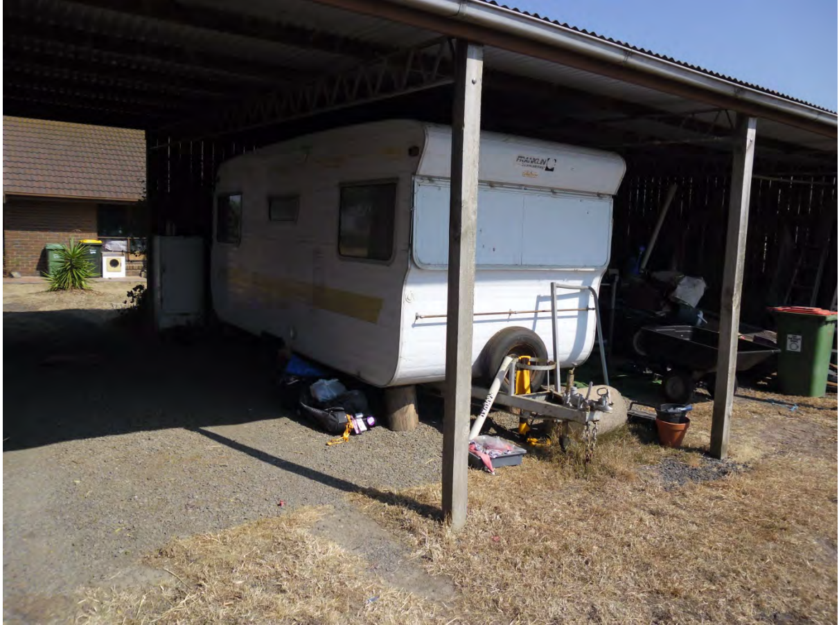
Photograph 33 – Carport at rear of house at 1990 Mickleham Rd (facing NW)
