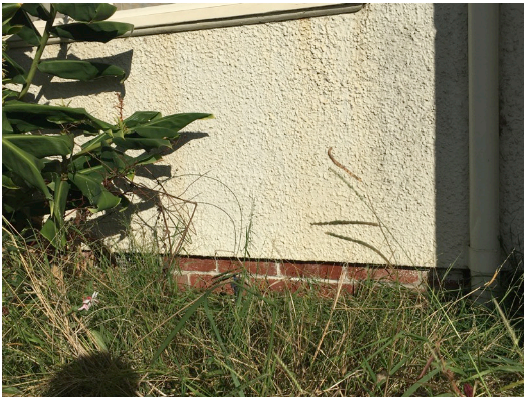
Figure 7: Detail of eastern façade – showing brick and roughcast render
