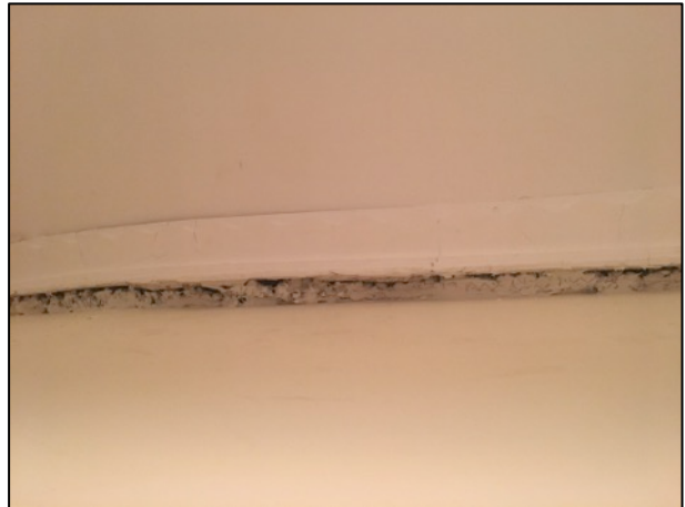
Photo N: Internal - water damage – western bedroom
