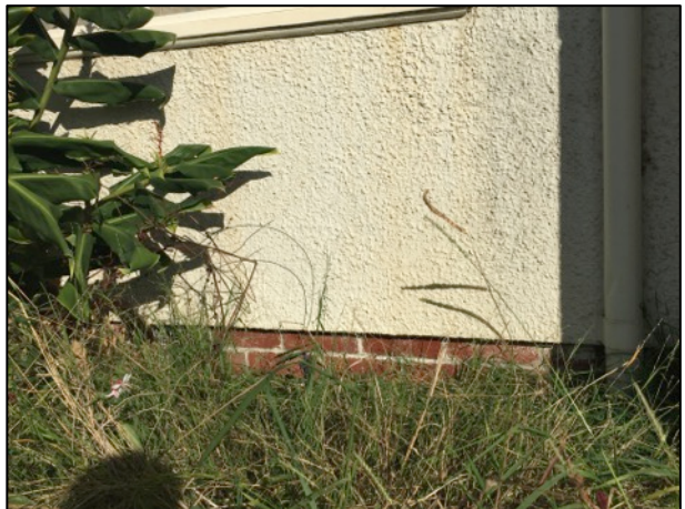
Figure 10: Eastern Façade – roughcast finish detail
