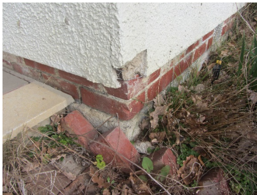
Figure 7. Concrete strip with two courses of red brick for providing base wall (Source: Context 2017)
