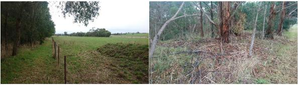
Inspection of the Deep Creek corridor revealed that it had been extensively modified by earthworks. This has comprised straightening the creek and channelizing it with the excavated soil placed in a low levee (up to 0.5 m high) parallel with and set back about five metres from the creek bank. This is shown in the photograph below.
