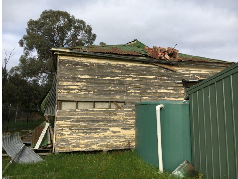
A side (west) elevation of the house. Weatherboards have been removed showing that the internal wall linings are asbestos/cement sheet (Photo: April 2018).
