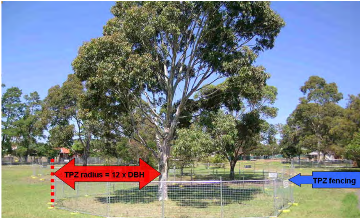
Figure 22: TPZ fencing is erected around retained trees prior to site works.
