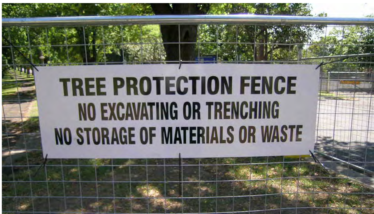
Figure 23: Example of a TPZ warning sign clearly displayed on TPZ fencing
