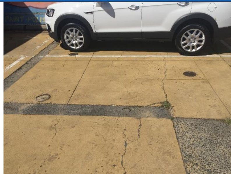
Plate 4 – Remnant UST fill points within Parcel 2
