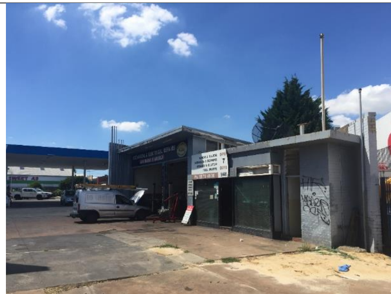
Plate 10 – Mechanical Workshop – Parcel 19
