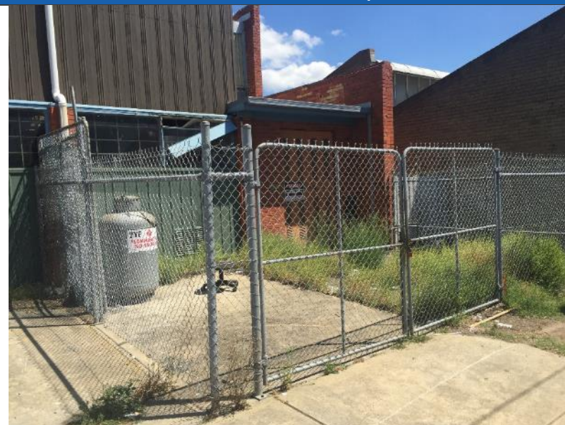
Plate 12 – Exterior of eastern portion of Parcel 15
