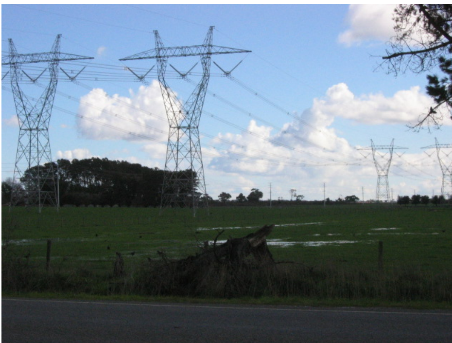
550kV Transmission towers and 66kV poleline through development area
