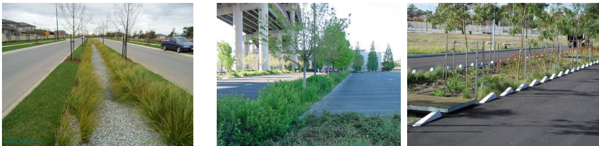
Figure 13 Different arrangements of kerbs with breaks to distribute inflow to bioretention swales
