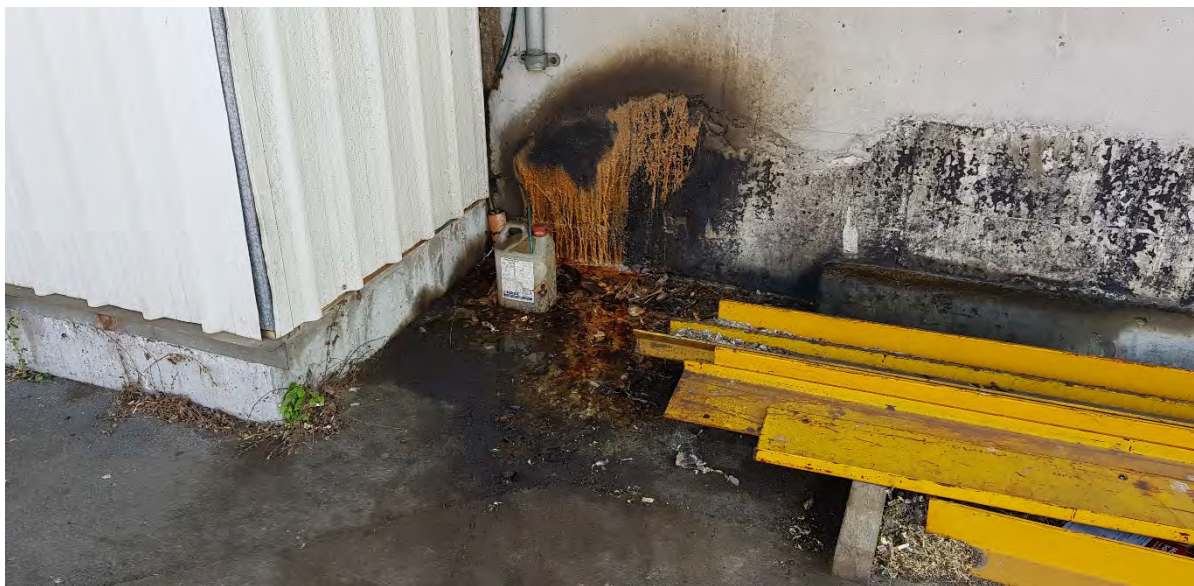
Photo 10. Oil on ground and wall on east side of main site building from compressor bleed valve.
