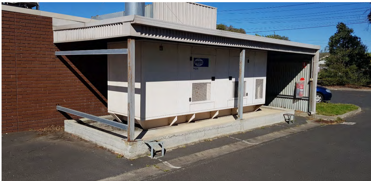
Photo 13. Diesel back-up generator.
