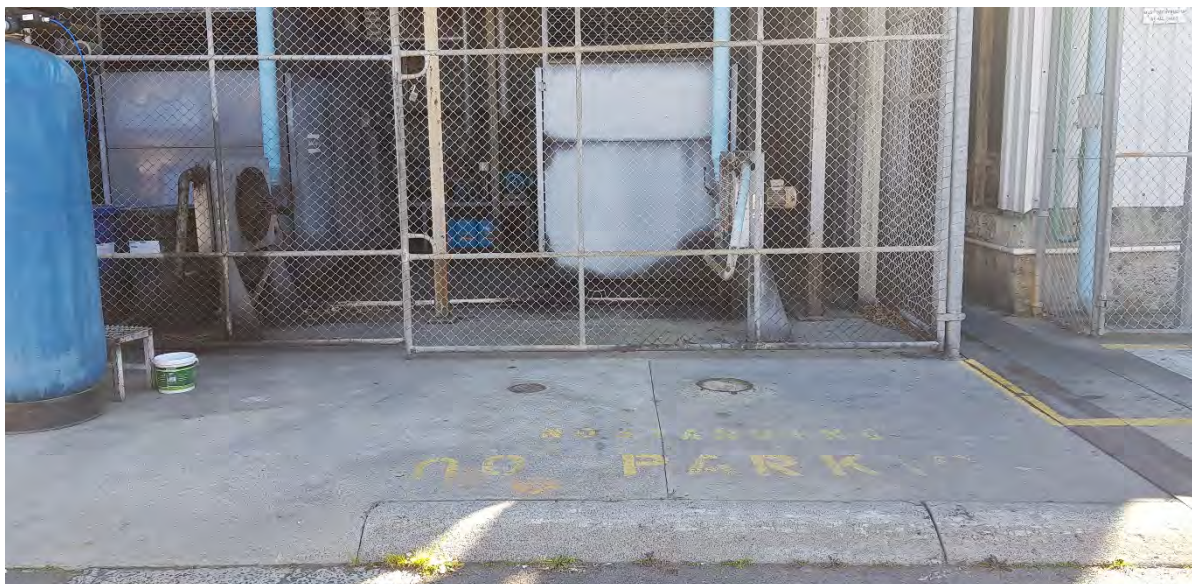
Photo 14. Fill points of decommissioned USTs south of compressor house.
