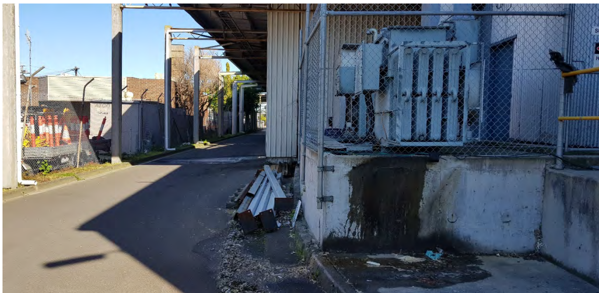
Photo 9. Staining on outside of transformer bund.
