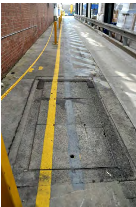
Photo 4. Triple Interceptor Trap east of pre-press (photo from Atma, 2012a).
