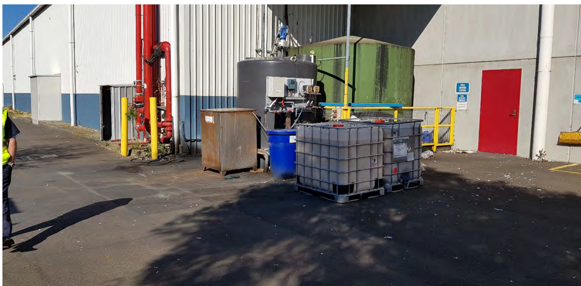
Photo 7. Trade waste ASTs, treatment and discharge area.
