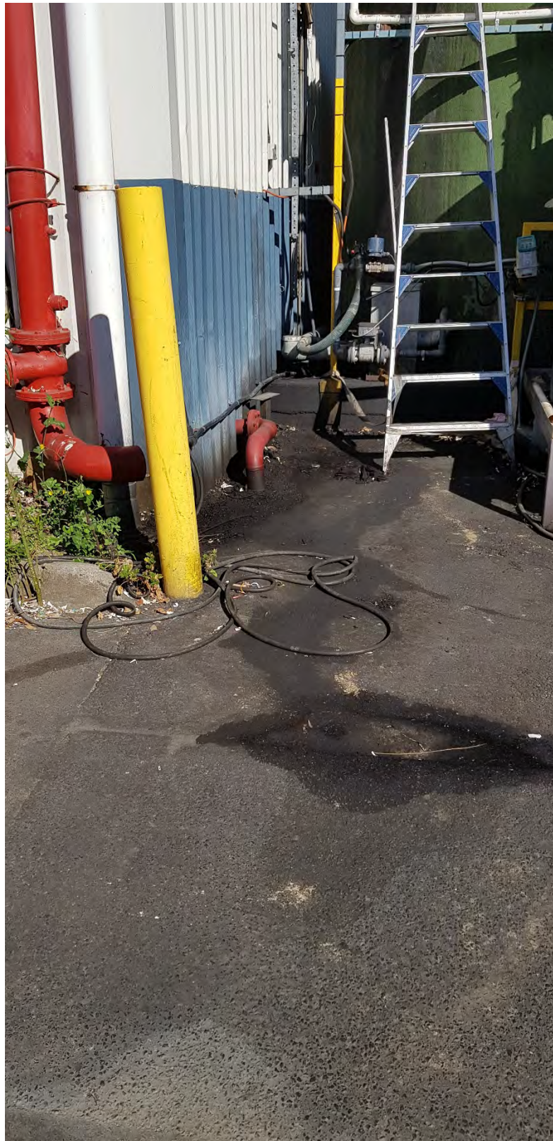
Photo 8. Staining on ground outside trade waste bund.
