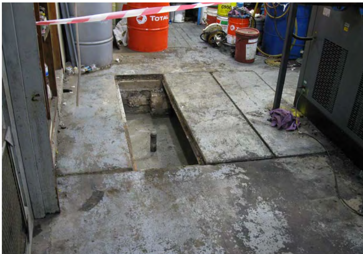
Photo 3. Decommissioning of UST within compressor house (photo from Atma, 2013).
