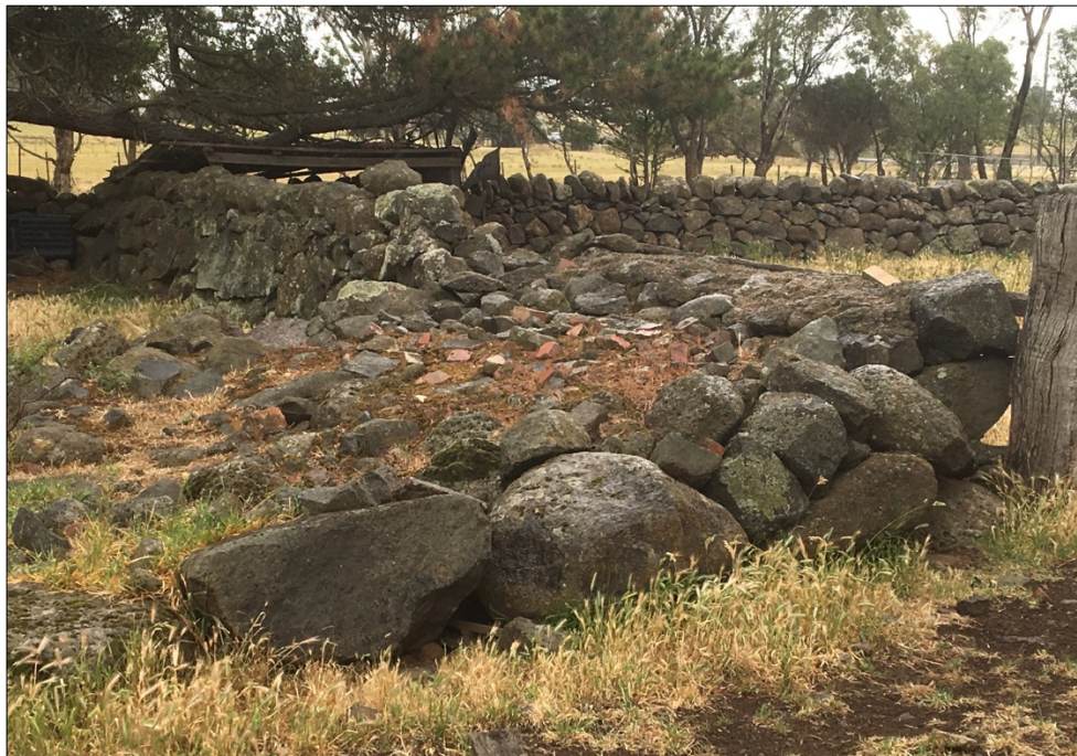
Figure 19 Remnants of the bluestone and brick stock ramp, south of the hay/machinery shed.
