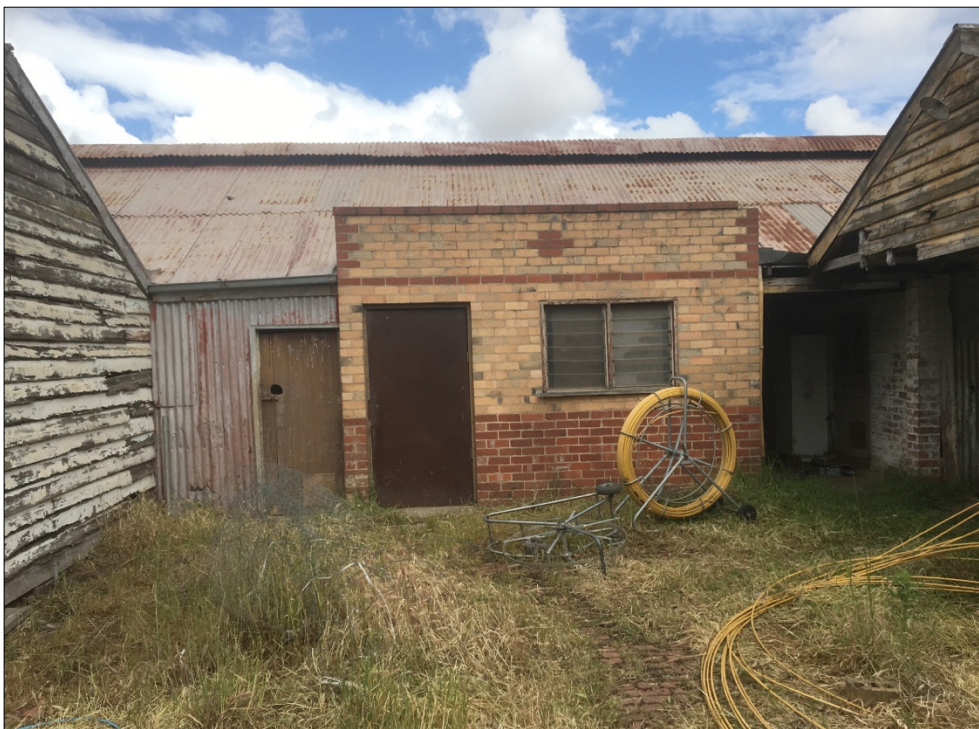
Figure 15 Part of the east elevation of the milking shed showing the postwar (?) addition.
