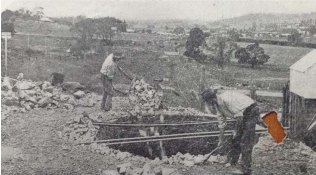
Figure 46 Top loading a pot kiln, 1906: view looking north towards Lilydale township Source: The Australasian , 7 April 1906, copy courtesy of Lilydale Historical Society
