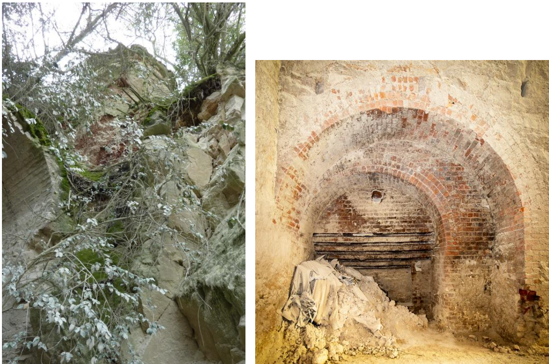
Figure 53 Left: Exposed shaft of c. 1880s pot kiln. Right: Base of a pot kiln in the Tunnel Source: Hin Lim (right)
