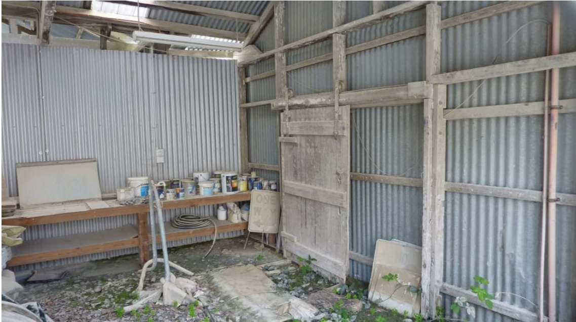
Figure 89 Top-hung timber door retained with the southern-most of the timber buildings to north of the Bacon Factory
