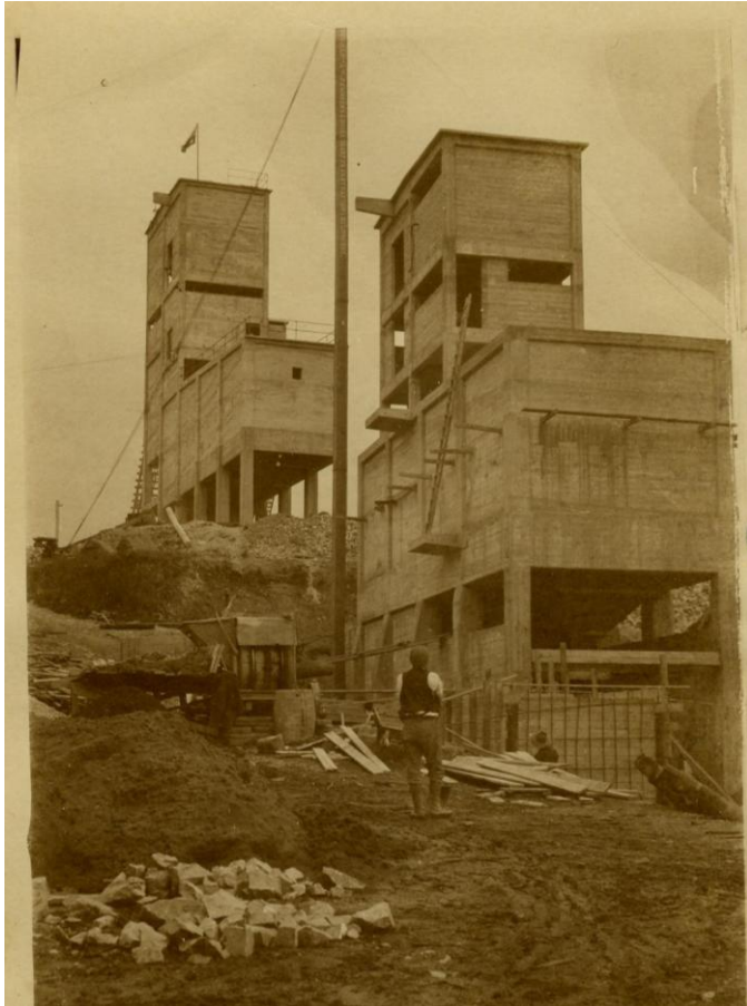
Figure 60 The Road Metal Plant (foreground) and Primary Crusher under construction, early-1920s Source: Yarra Ranges Regional Museum
