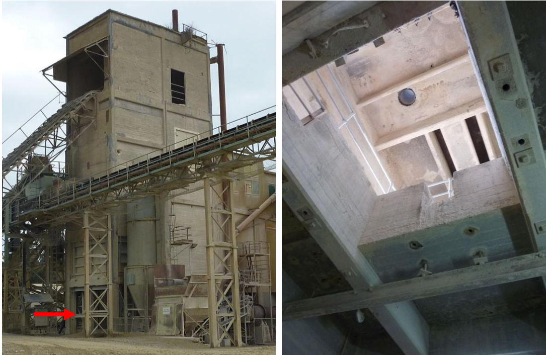
Figure 65 Left: South and east elevations of the Picking Station; the modern structural support is indicated; Right: Double-height space at the top of the Picking Station
