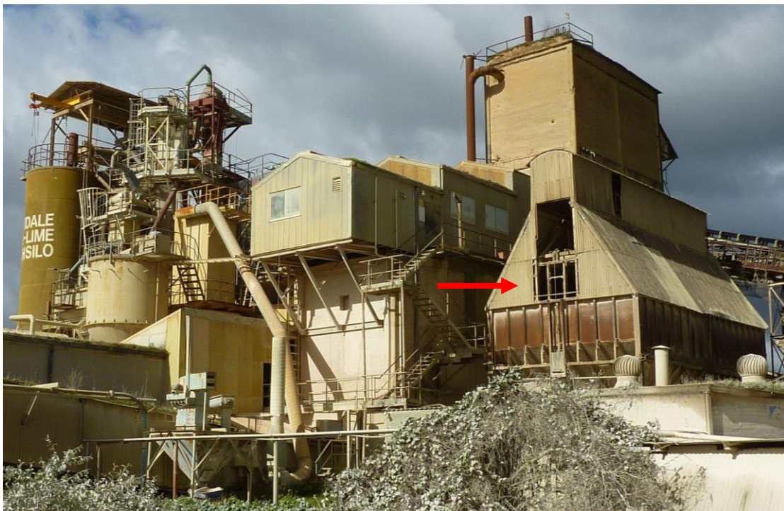
Figure 70 View of the Picking Station (at top right) from the north: note the accretions and additions, and the riveted steel hopper to the right of picture (indicated)
