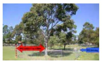
Figure 8: TPZ fencing is erected around retained trees prior to site works.
