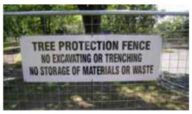
Figure 9: Example of a TPZ warning sign clearly displayed on TPZ fencing.
