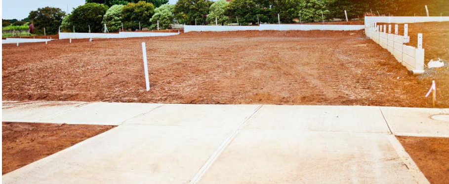
Figure 15: Lot has been graded or benched with a combination of retaining walls and lot grading to ensure a flat building pad is provided
