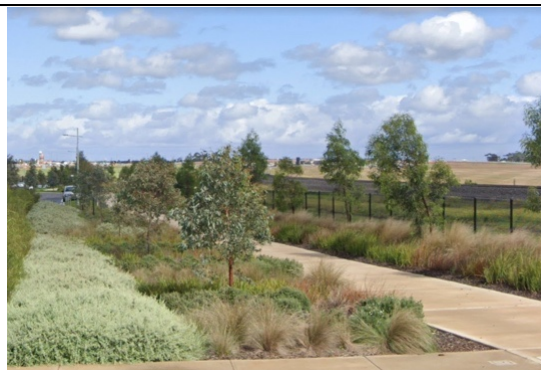
Aylesbury Avenue interface to rail features a shared path and vegetated WSUD swale treatment
