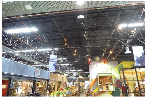
New specialty section - north-west end Space frame widely visible
