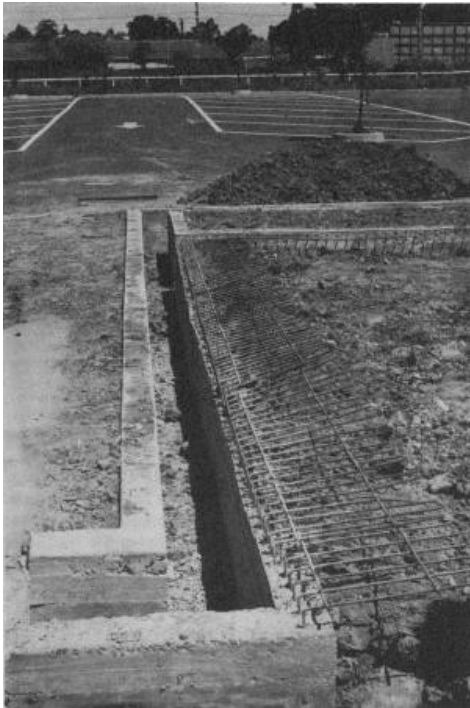
Socket/slot foundation for cantilevered walls (1969-70) (Source: 'Preston Market', Foundations , no. 70, p10)
