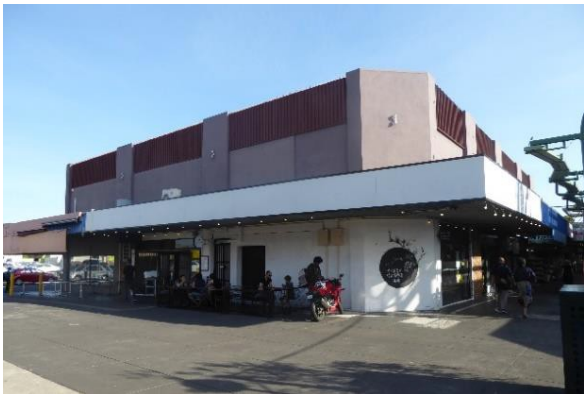
Original shops (pre and post-1970), north-east, now rendered with Kliplok to parapet
