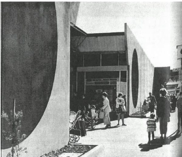
Original wall finish (Mary Street) with painted circles Note garden beds (Source: B Crisp, 'Tilt-up Construction in Australia', Constructional Review , Nov. 1970, p58)
