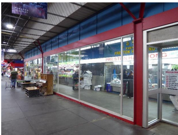
Full height glazing to food hall, highlights painted blue Original concrete, square pattern
