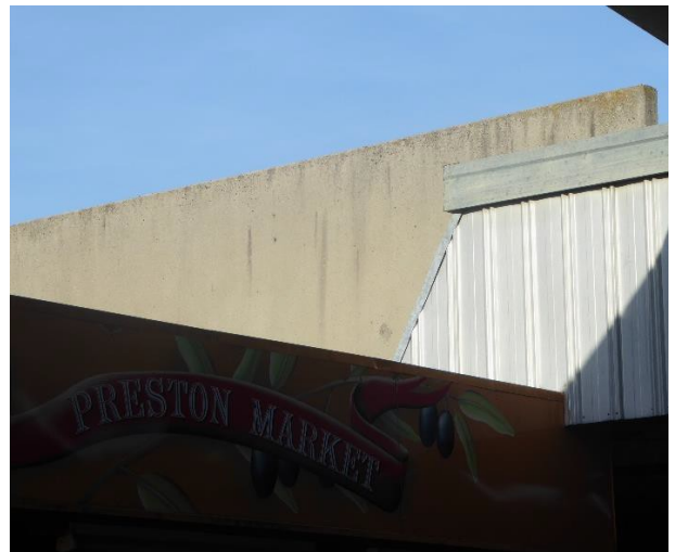
Section of original unpainted, sand-blasted concrete Adjacent is the original metal fascia
