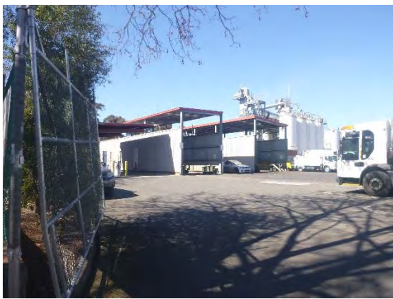
Photo 15. Property 61, Citywide asphalt plant, with wash bay, six (6) fuel bowser and a fleet servicing area
