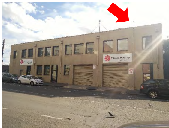
Photo 27. Property 219, vent pipe indicates potential for a UST or former UST to be present at site
