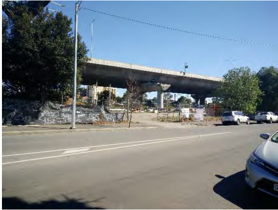
Photo 13. Property 59, cleared and used as construction depot/storage
