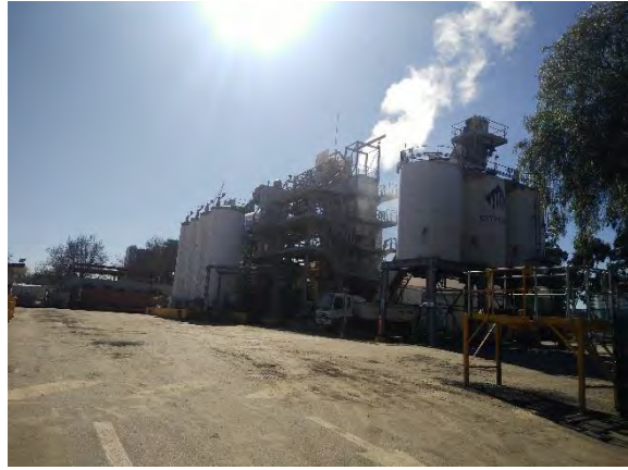
Photo 14. Property 61, Citywide asphalt plant
