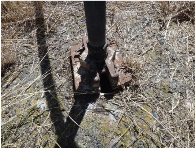
Windmill bore BH17. Surface water can readily enter the well
