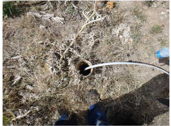
BH16. Former windmill bore no longer sealed
