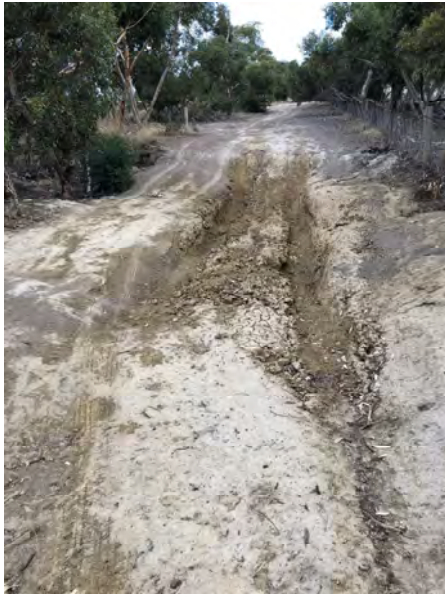
Figure 4-3 Significantly eroded sections and inundations at low points along the path
