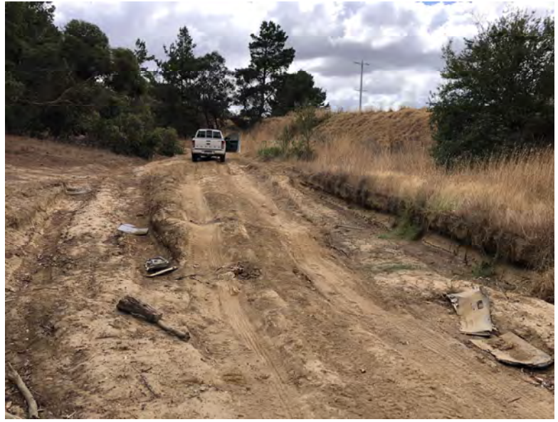
Figure 4-3 Significantly eroded sections and inundations at low points along the path
