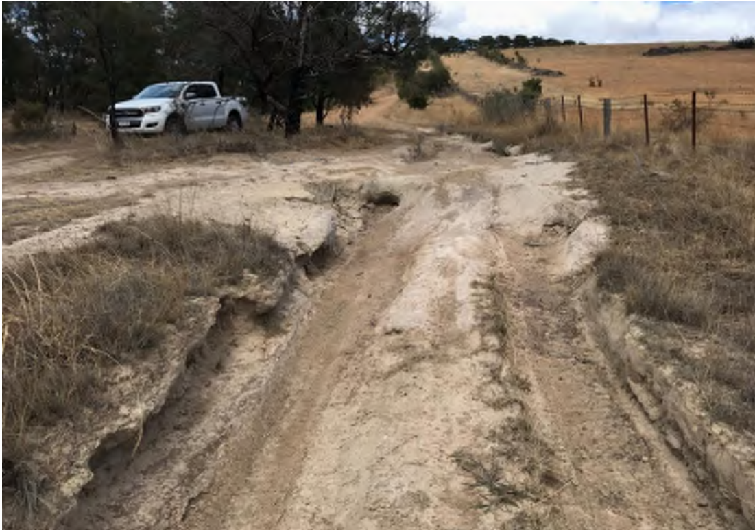
Photograph 7-9 Erosion on the unsealed track
