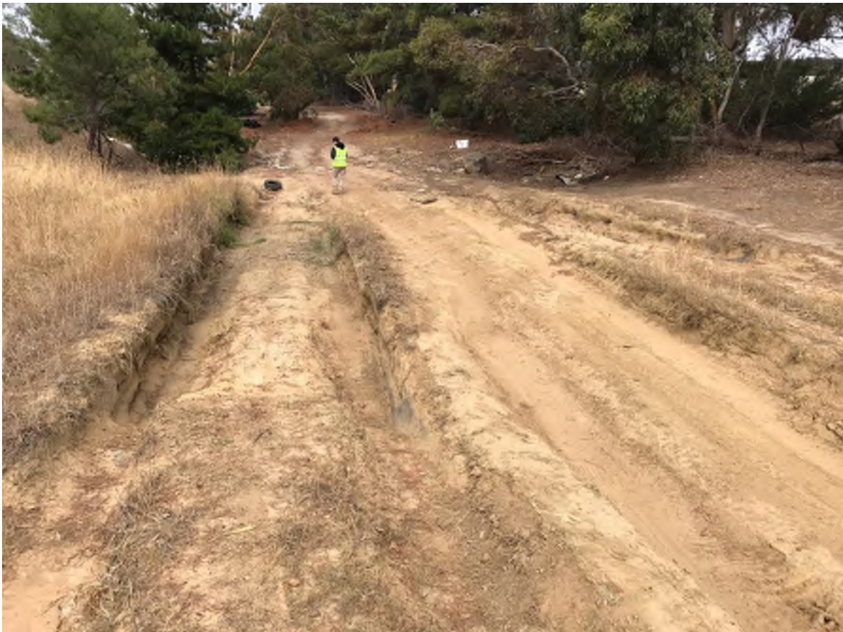
Photograph 7-2 Erosion on the unsealed track adjacent to an existing culvert and a natural low point
