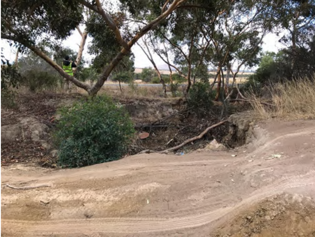
Photograph 7-15 Erosion on the eastern edge of the unsealed track at a natural low point and an existing culvert
