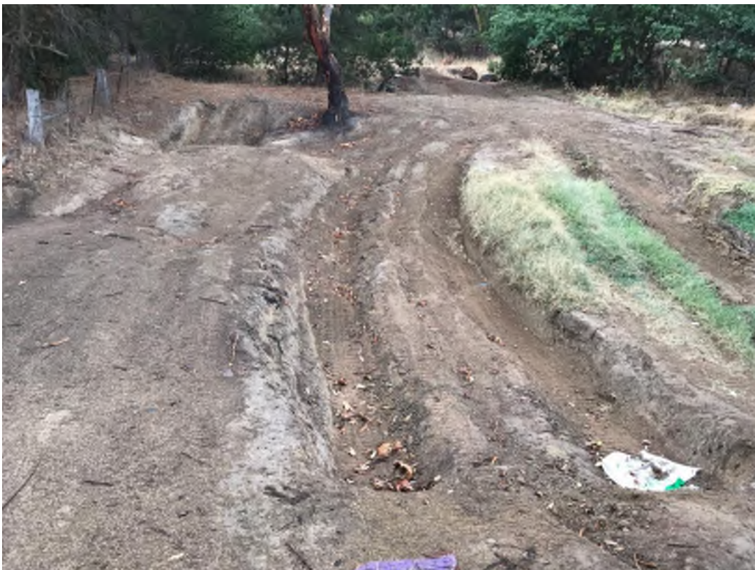
Photograph 7-6 Erosion on the unsealed track adjacent to an existing culvert and a natural low point
