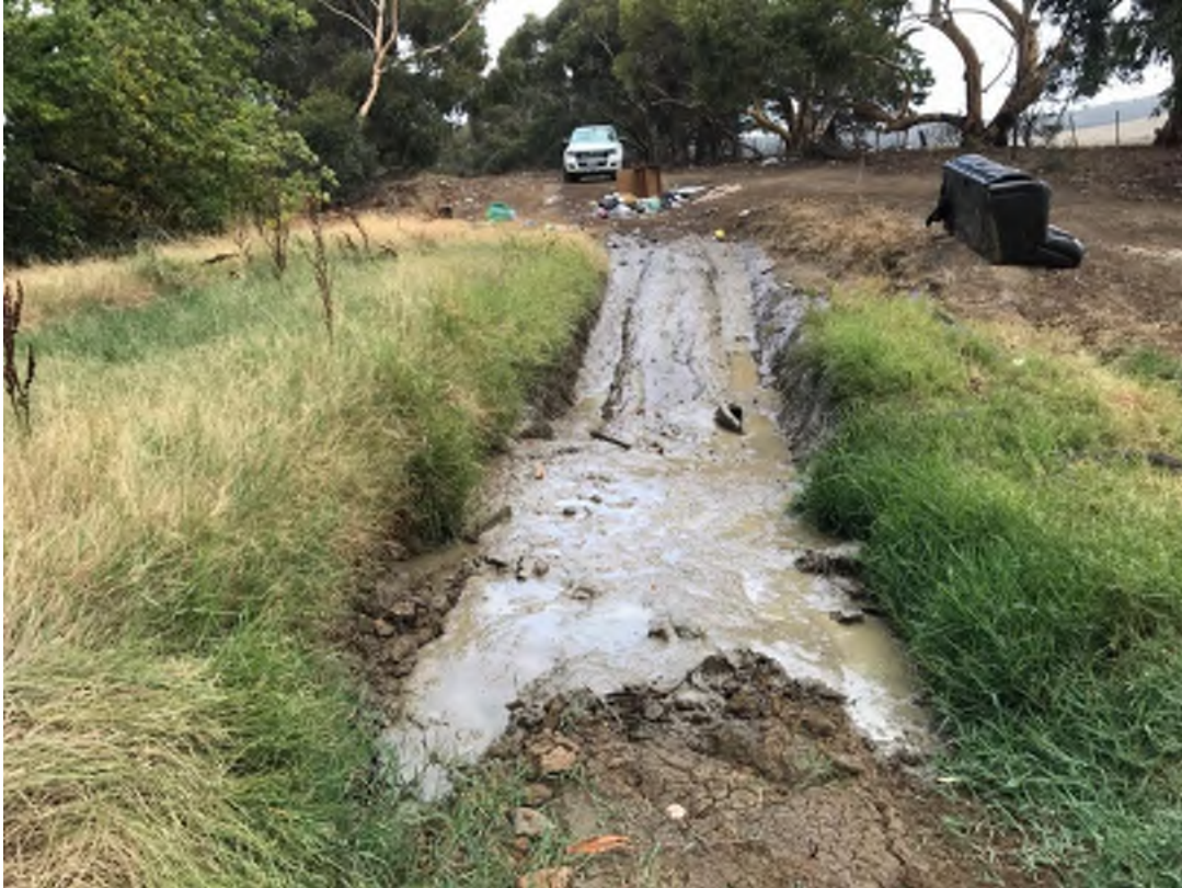
Photograph 7-7 Wet soil material observed as a result of ponding water in the eroded area
