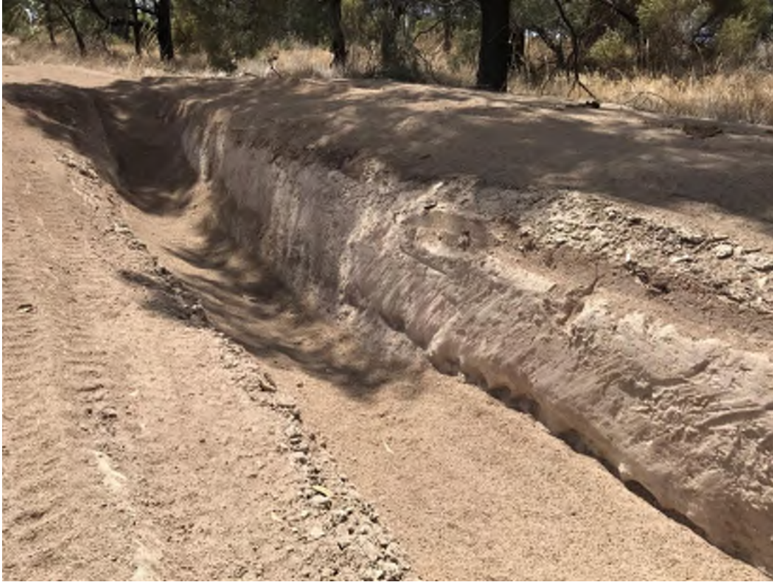
Photograph 7-11 Erosion on the unsealed track
