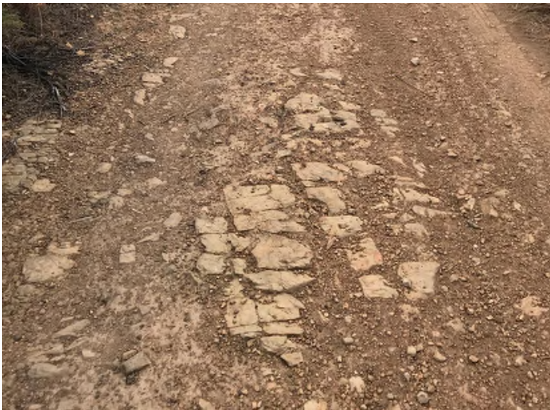
Photograph 7-8 Siltstone observed at the surface of the unsealed track
