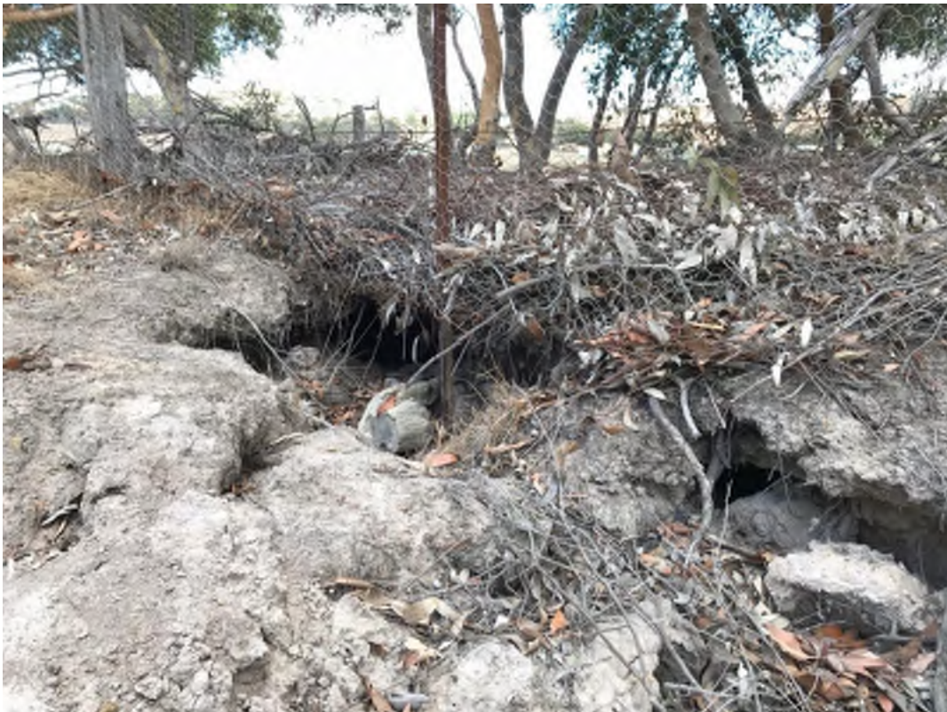
Photograph 7-14 Tunnel erosion on the western edge of the unsealed track at a natural low point and an existing culvert
