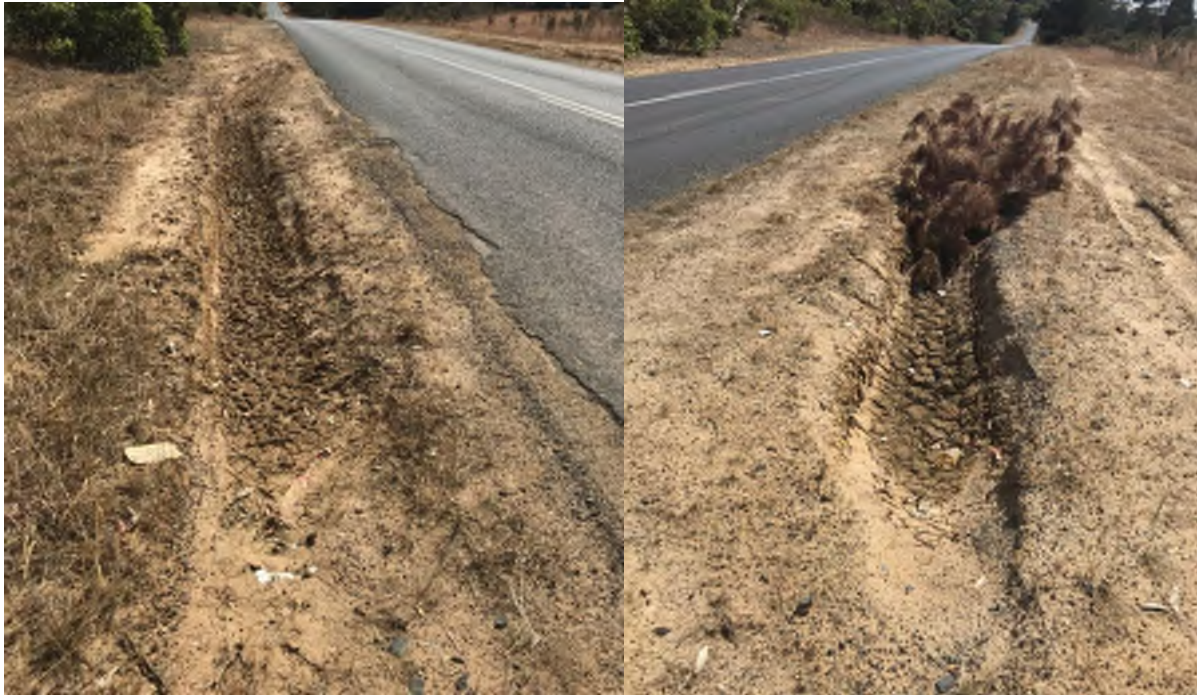
Photograph 7-1 Erosion adjacent to Old Sydney Road Pavement at Intersection IN-18 (looking north)
