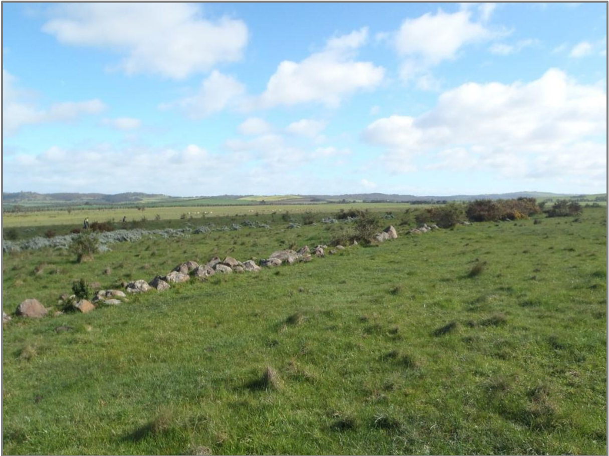
Figure 15: Dry stone wall in extremely poor condition within property 7
