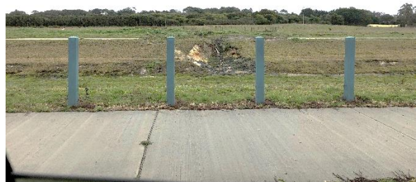
Existing headward and gully erosion along the newly constructed waterway banks from DETV land
