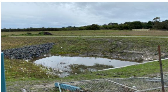
Powlett Ridge Estate temporary sediment basin, looking upstream of constructed waterway 'west' alignment.
