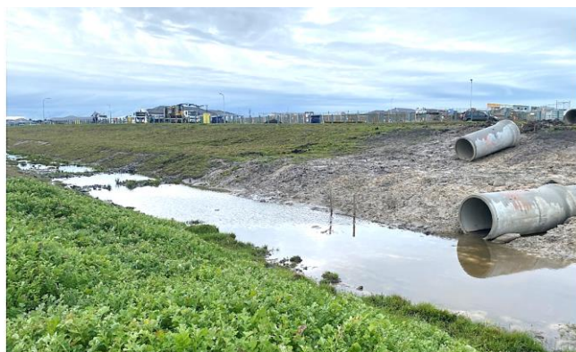
Existing outfall drain from Powlett Ridge estate into constructed waterway 'west' alignment.
