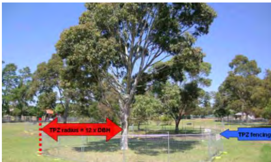
Figure 25: TPZ fencing is erected around retained trees prior to site works.
