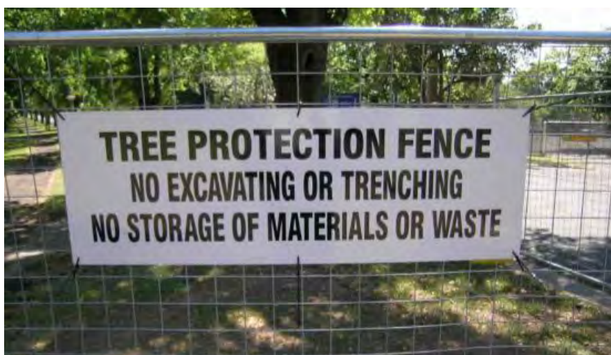
Figure 26: Example of a TPZ warning sign clearly displayed on TPZ fencing.
