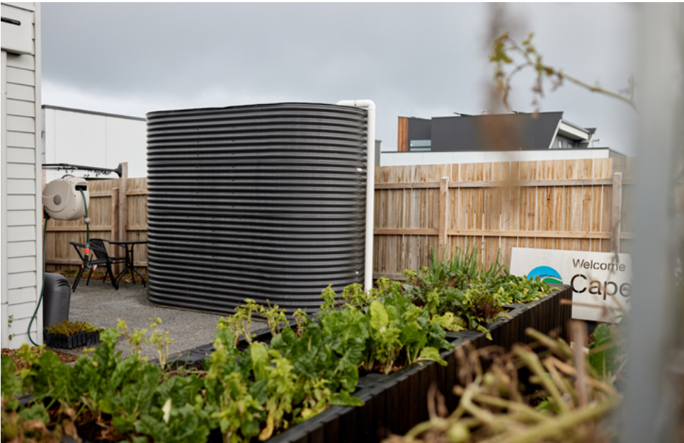
On-lot rainwater tanks can reduce stormwater flows (lessening damage to local waterways), while also providing alternative water sources for uses such as landscape and garden irrigation. Image by Kim Landy
