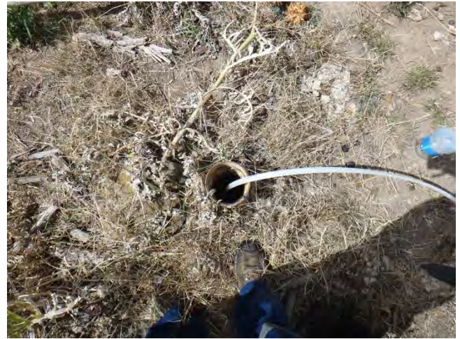
BH16. Former windmill bore no longer sealed
