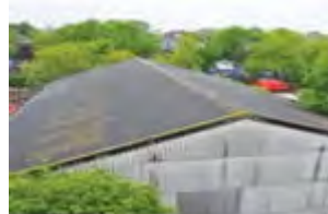
AC roof and wall cladding (non-friable)
