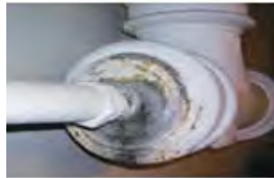
Amosite and chrysotile packing on a water pipe (friable)
