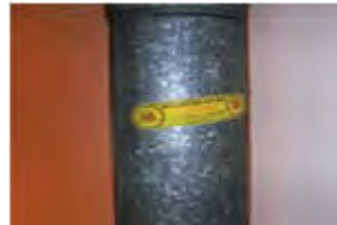
Metal clad gas Flue containing chrysotile lining (non-friable)
