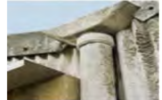
AC downpipe (friable)
