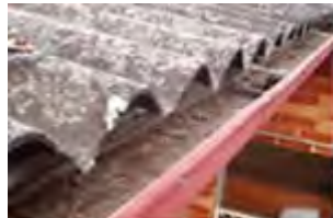
AC moulding gutter (friable)
