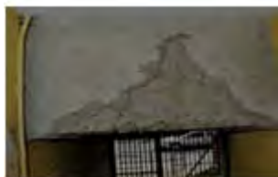
Spray coating on a building walkway (friable)
