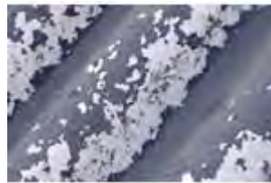
Friable asbestos roof cladding (friable)
