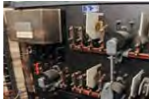
Open electrical switchboard with asbestos flash guard (non-friable)
