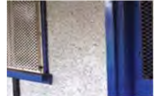
Chrysotile pebble dash exterior wall coating (non-friable)
