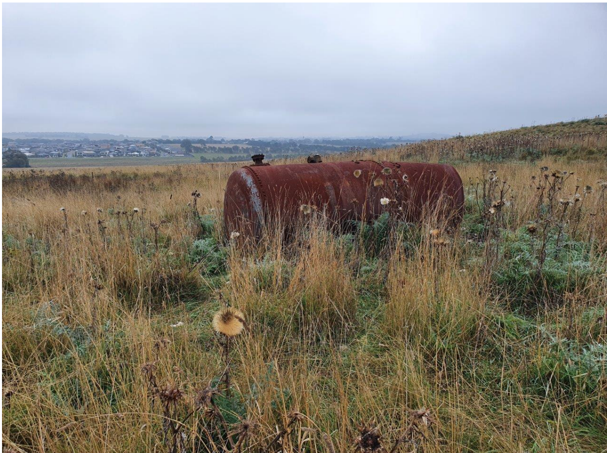
Photograph 14: View of a disused fuel storage / boiler tank in the eastern portion of the site. The tank was empty and open on one side.
