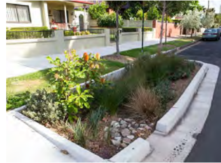
Household driveways and roofs connected to raingardens
