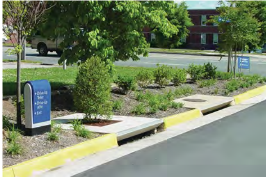
Passive street tree irrigation
