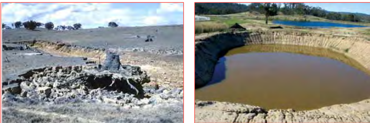
Figure 4.1 Tunnel erosion of dispersive clay subsoil, https://vro.agriculture.vic.gov.au (accessed 2022) (Left), and construction of dam in dispersive soils leading to rill erosion, https://nre.tas.gov.au (accessed 2022) (Right)
