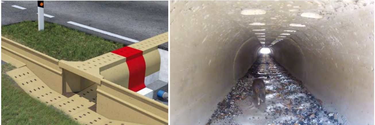
Figure 3.3 Culvert underpass design implemented at RBGC (left), with Southern Brown Bandicoot shown using the culvert (right).
