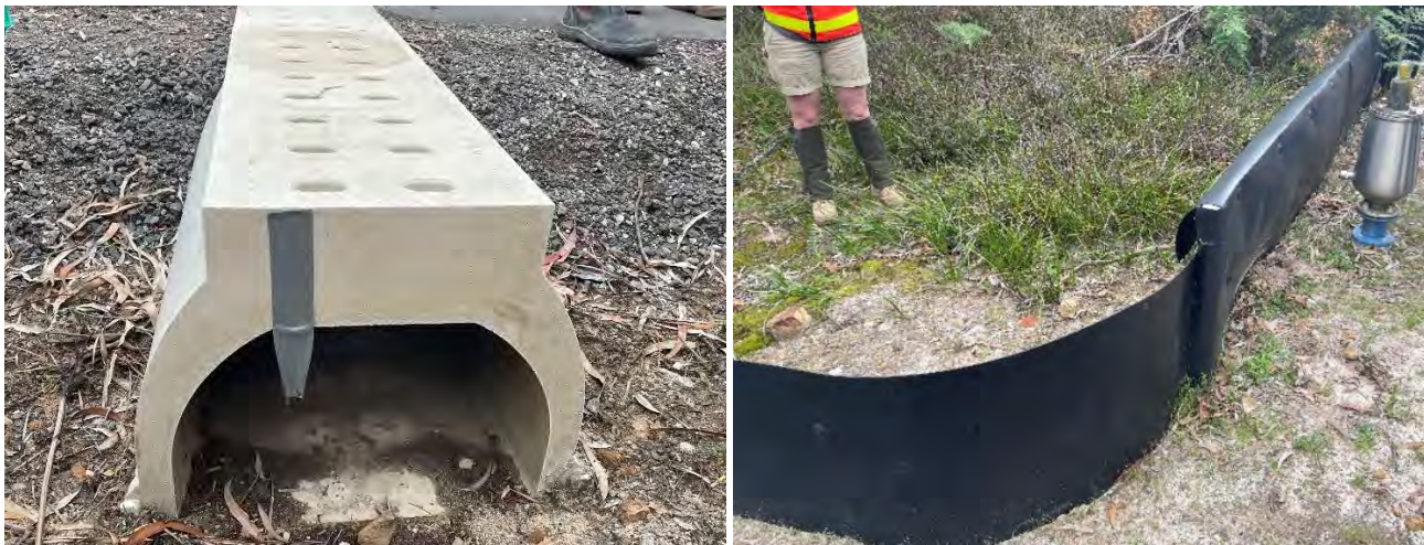
Figure 3.4 Culvert installed at RBGC (left) with lightwells visible in the roof of the culvert. Wildlife-exclusion fencing (right), which includes habitat-facing floppy overhang to deter wildlife from crossing.
