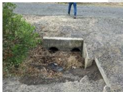
2 x 350mm dia. pipes
