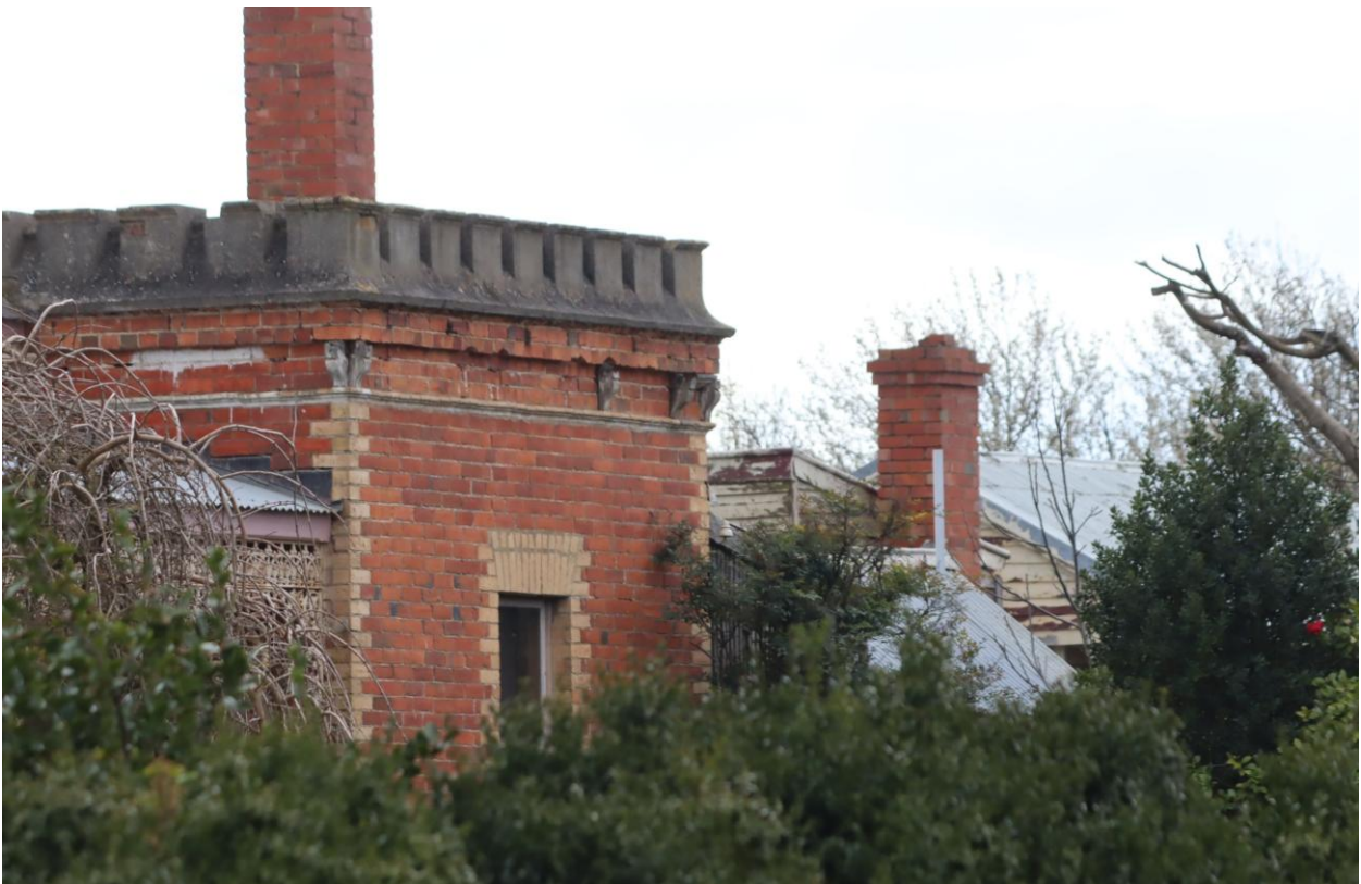
Close-up of eastern crenelated parapeted bay (replacement Federation-era chimney evident). Note missing bracket. (Source: RBA, August 2024)
