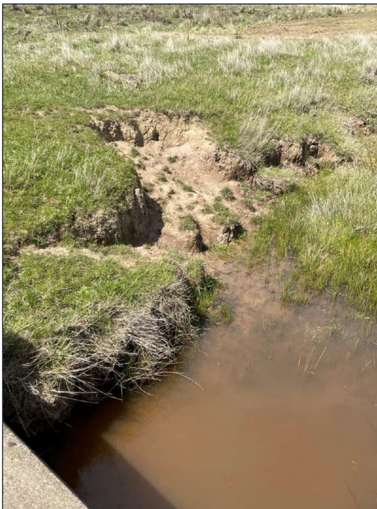
Figure 3-17 Local Erosion on the right bank of the Unnamed Drain
