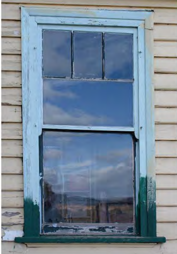
Figure 12 Window west elevation 75 Browns Lane, thought to be the original window form generally
