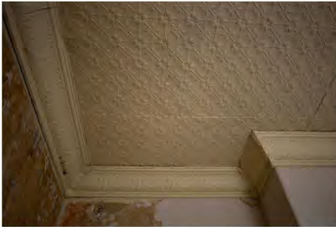
Figure 43 Kerr's farm house, room 1- pressed metal ceiling and cornice
