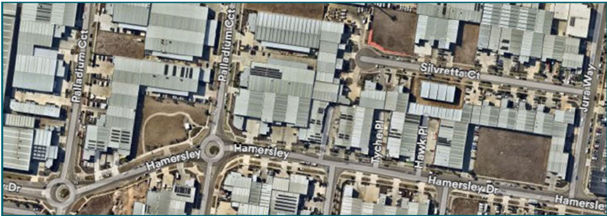
Figure 12: Clyde North industrial precinct Note direct access to key routes & parking at property frontages Nearmap 4/3/2025
