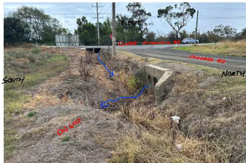
Figure 4 - Ex. Outfall in Moores Rd (looking West)
